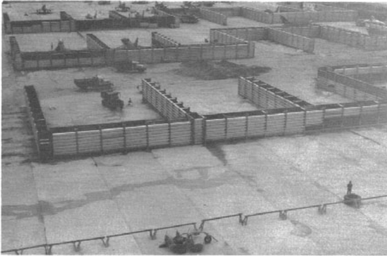
After the Viet Cong made the wide open spaces untenable, Army Engineers began constructing hundreds of these revetments at Bien Hoa AB. (top) (USAF) 481st TFS Hun begins pull-up after release of 750 lb. bomb. (right) (USAF via Dave Menard)
