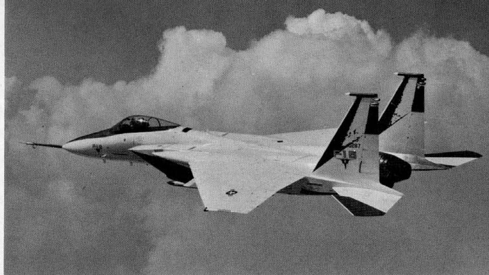
**The F-15 Eagle has been flown up to 9.0 Gs during flight testing at Edwards AFB, Calif. The pilot said the airplane had excellent and stable handling under these conditions. (McDonnell Douglas)**
