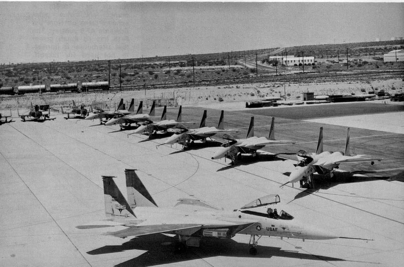
Aircraft #1 (10280) taxis in front of six F-15s and three F-4s at the USAF Flight Test Center, Edwards AFB, Calif. Note that five of the F-15s have the test "pitot boom" installed on the nose. The remaining two have the production type radome. The F-4s are used as high speed chase aircraft during testing. (McDonnell Douglas)
