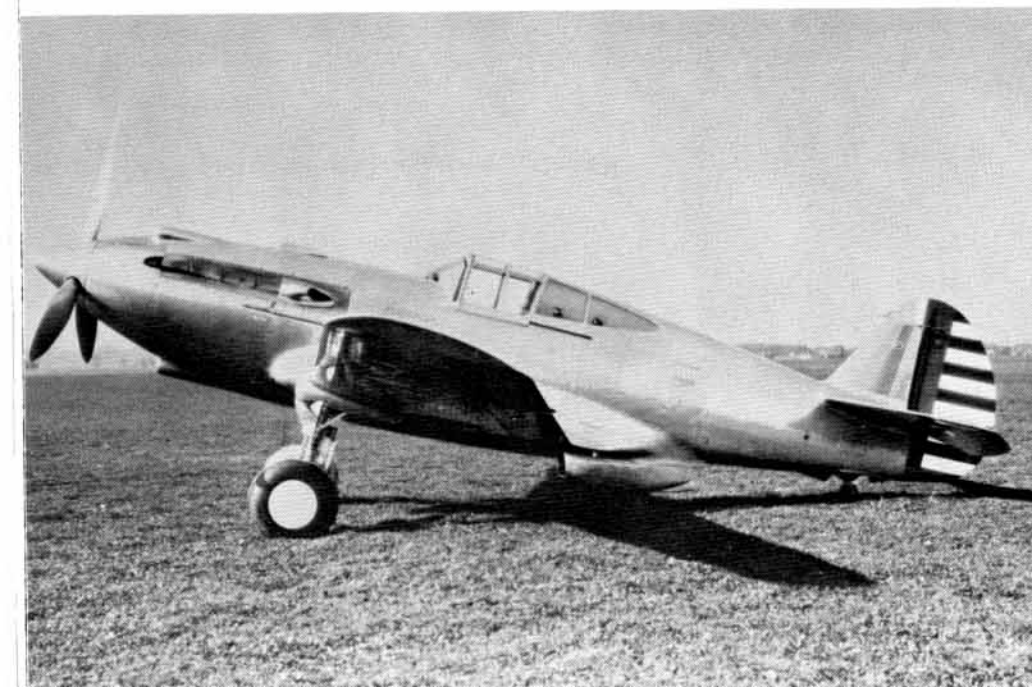
The XP-40 Prototype, Air Corps serial number A.C. 38-10. Designer Donovan R. Berlin elected to locate the scoop for the radiator under the belly, but fear that it might be damaged by debris thrown up by the slipstream on takeoff and landing led to its relocation. Berlin was later proven correct when the North American P-51 flew with the radiator in the same location. [USAAF]
