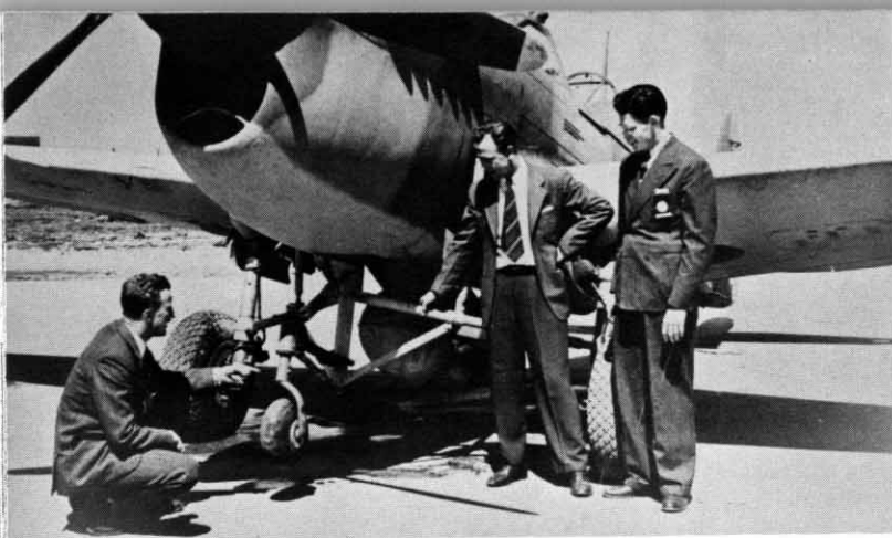
Officials of the Buffalo, New York plant took over "Susie Q" which had been modified to include twin cockpits, dual controls and a tricycle landing gear to train ground crew mechanics how to taxi and move an aircraft under its own power from one location to another. This P-40K had been rendered unflyable. [USAF]
