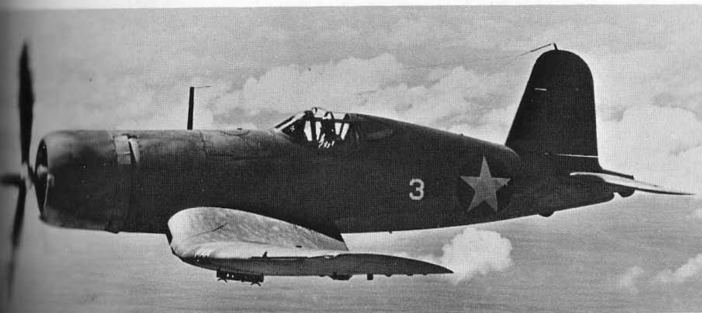
F4U-1 and F4U-1A Corsairs from MCAS Cherry Point. To compensate for the additional weight added by changes from the XF4U-1, Vought installed a P&W R-2800-8 engine with 2,000-HP for take-off. October 1943. [National Archives]
