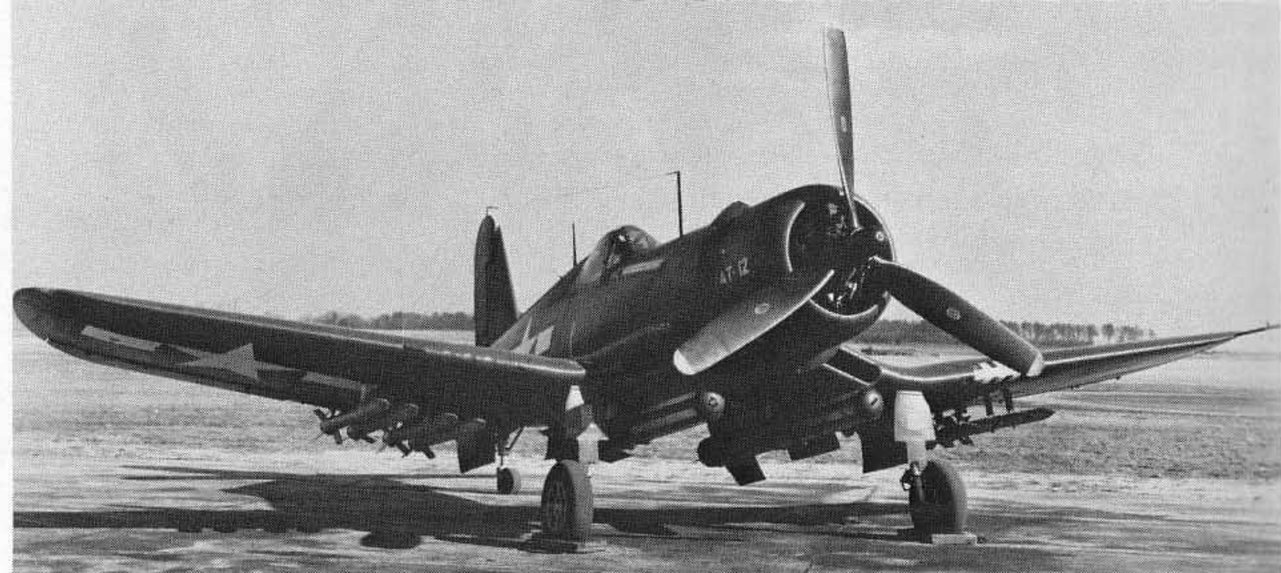
Fully loaded F4U-1D [57369] with 8-HVAR and 2 "Tiny Tim" 11.75-in. rockets, the largest rocket to be used by the U.S. during WWII. Tiny Tims packed 152-lbs. of TNT in the warhead and were essentially rocket-powered flying 500-lb. bombs. In mid-1944 a plan known as "Project Danny" to the Marines was formed to assign MAG-51 Corsairs the objective of attacking German V-2 rocket launching bases with the "Tiny Tims" but "Danny" never happened as the delays with the new weapon forced the U.S. and British Infantry to do the job, January 31, 1945. [National Archives]
