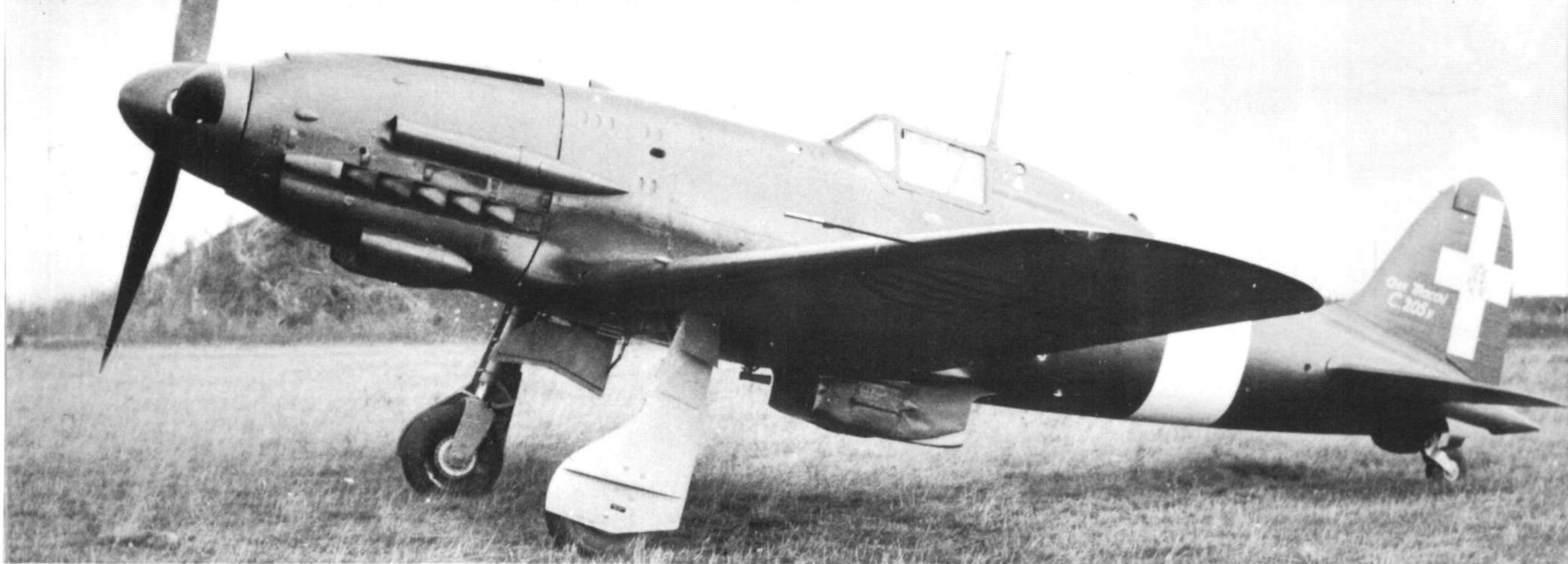
The C.205V ( Veltro -Greyhound) prototype, showing the twin cylindrical oil coolers, blunter spinner and retracting tailwheel, at the Guidonia Test Center.
