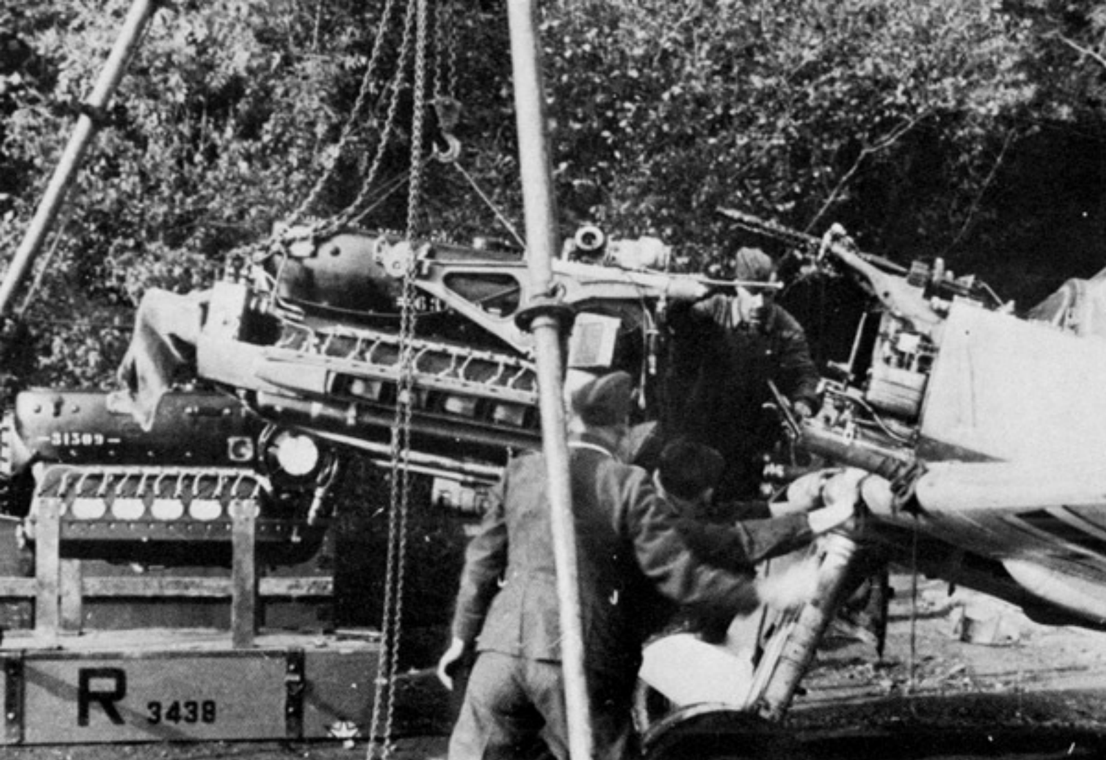
Even under the severely primitive conditions that existed in the Balkans, the 'blackbirds' could quickly change an engine. (Obert)
