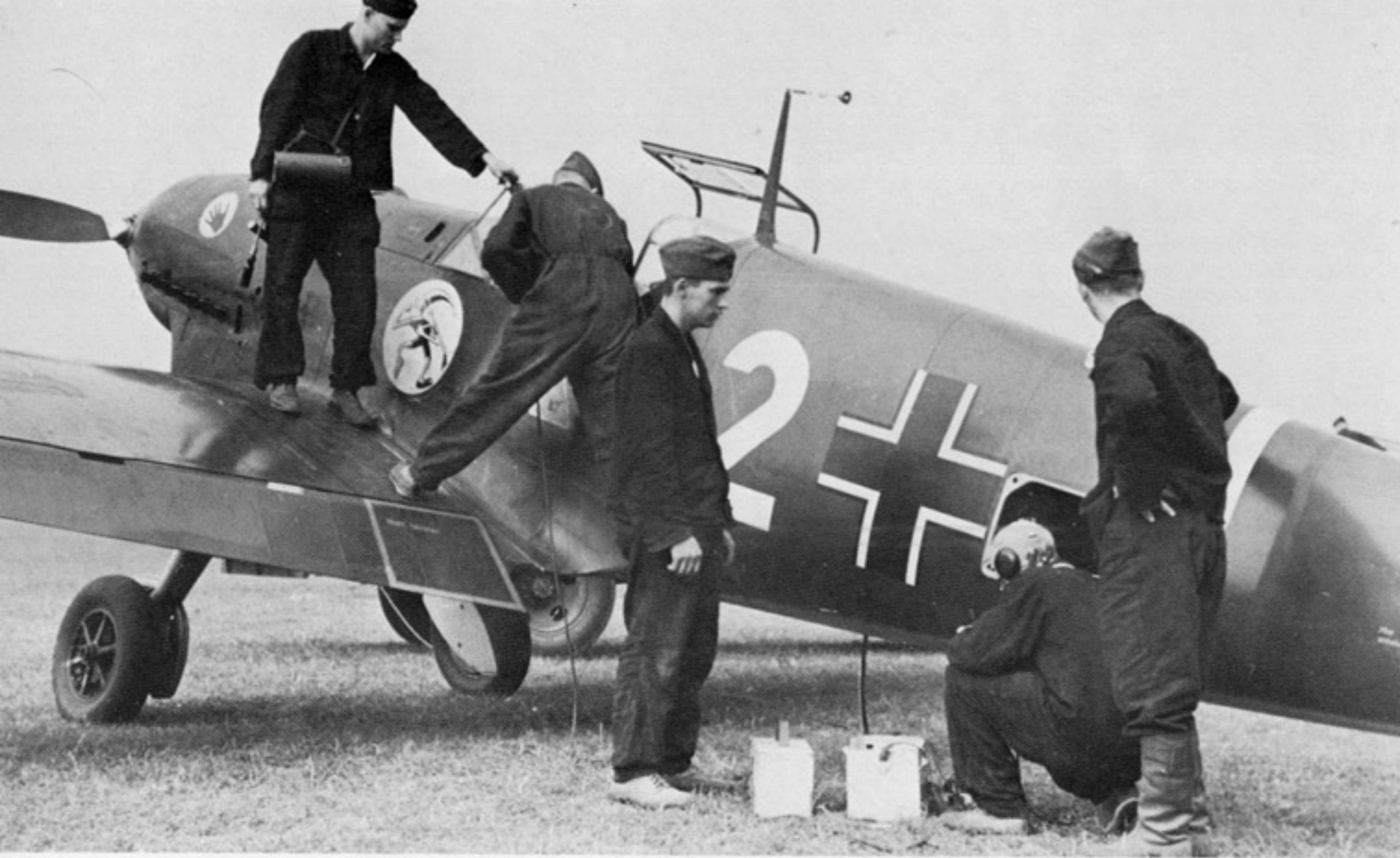
'White 2' of I/JG 137 undergoing radio tests. Note how the 'blackbird' on the wing is carefully avoiding the red outlined 'No Step' area on the flap. The significance of the white band is unknown. He 51-equipped Geschwadern used a white band to denote the second Staffeln in each Gruppe but since only one machine is so marked, this probably is not the case. The band may have denoted the Staffelkapitän's machine. (Bundesarchiv)
