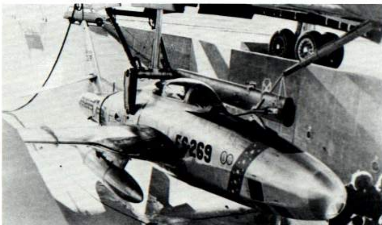
A 91st SRSq RF-84K production FICON aircraft in the pit at Fairchild AFB. The aircraft is being prepared for loading into the open bomb-bay of a B-36 mothership. Another method of loading the RF-84Ks into the B-36 mothership was by backing the GRB-36D onto a large set of ramps which elevated the bomber's fuselage high enough to clear the RF-84K's vertical tail. (AFM)
