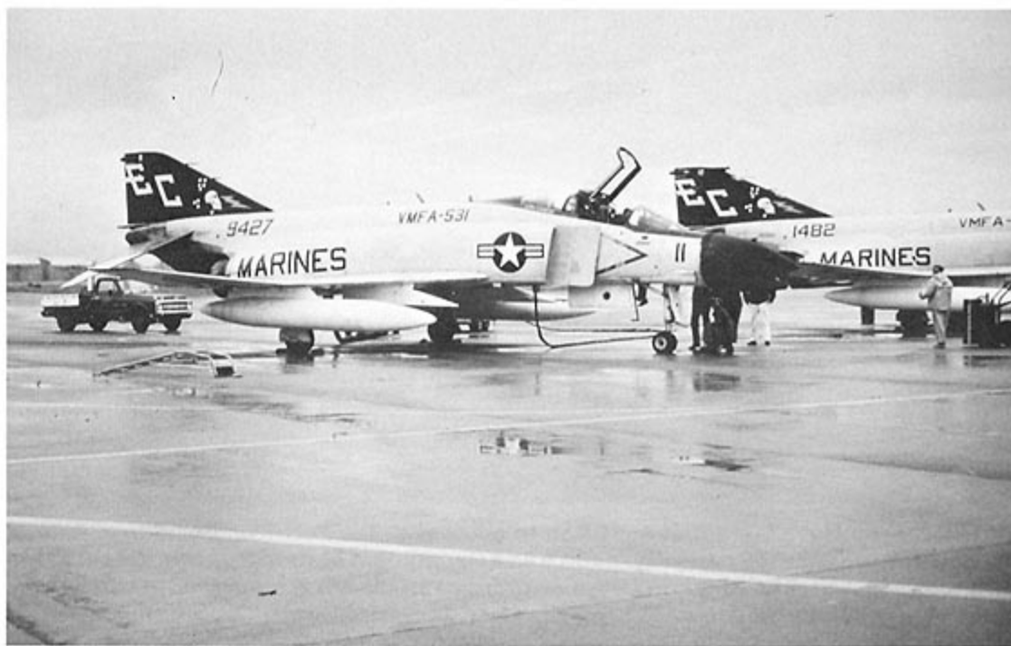
(Above) A VMFA-531 "Gray Ghosts" F-4B on the ramp at McChord AFB in 1971. The tail and wingtips are Black with White trim and a Yellow lightning bolt. The second aircraft has been fitted with the fincap leading edge APR-30 RHAW antenna. (Brewer)
