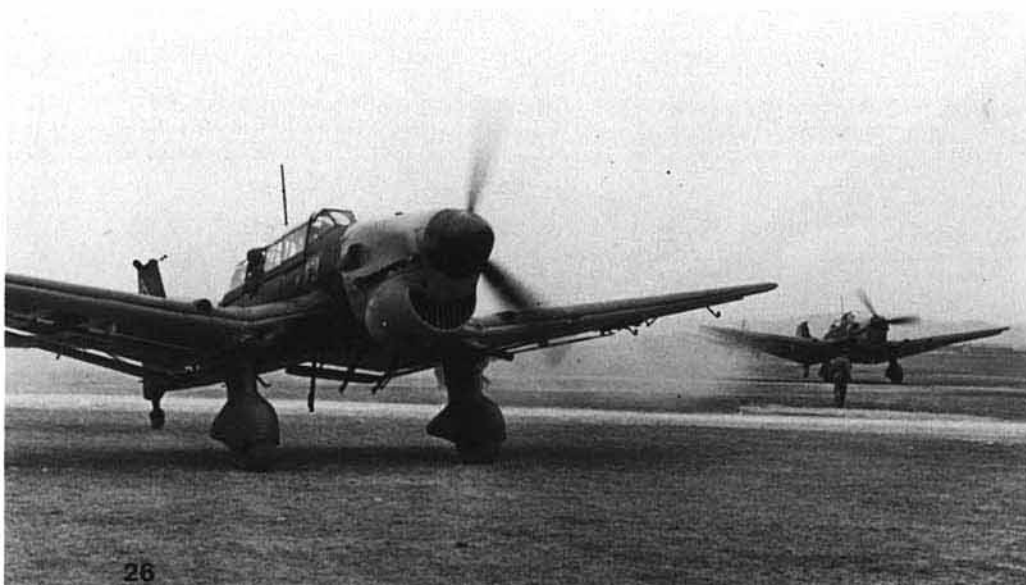
(Above) The undercarriage siren, cowl, and stencil markings can be appreciated here, including the small manufacturer's data plate just forward of the wing root. The Yellow, Red and Black shield of Stab/II/St.G 77, which saw action in the Balkans and Mediterranean during the early months of 1941, is carried below the windscreen. (Bundesarchiv)
