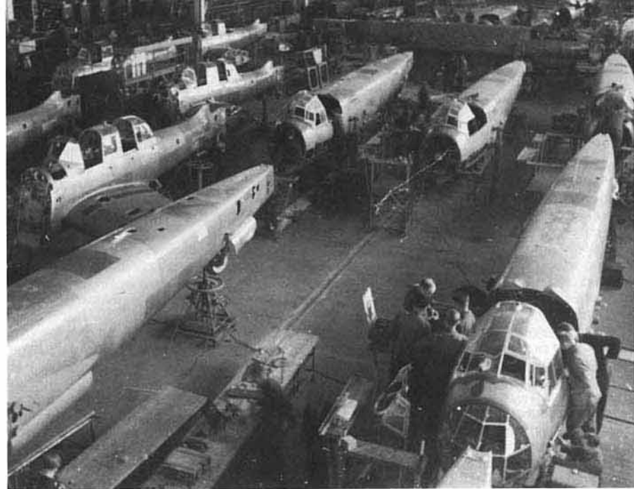
(Above) Ju 87B-1s sharing an assembly line with Ju 88A-1 medium bombers during 1939. In time the Junker's assembly lines at Berlin-Tempelhof and Bremen-Lemwerder would become responsible for the bulk of Ju 87 production, with only some 430 examples being manufactured at the Junkers' Dessau facility. (Bundesarchiv)
