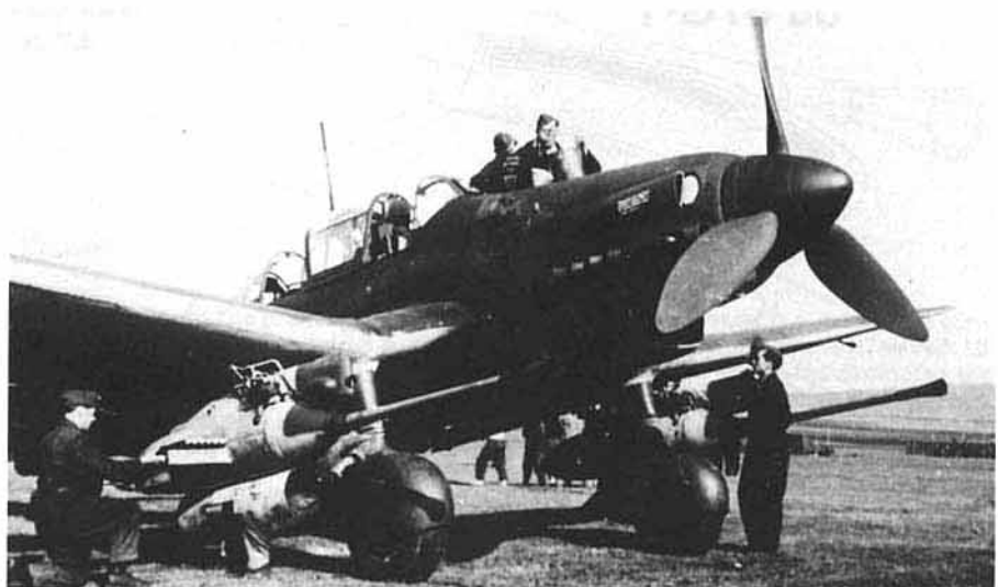
(Right) Produced in greater numbers than the Ju 87G-1, the re-built Ju 87G-2 was based on the long wing span Ju 87D-5 and was a much cleaner aircraft; all traces of the underwing dive-brake mounts and light caliber wing guns being deleted. For access to the cannon mechanism, the side panels of the cannon pods were hinged to fold downward and the end caps were removable fore and aft. Cannon installations were the same for both the G-1 and G-2. (Hans Obert)
