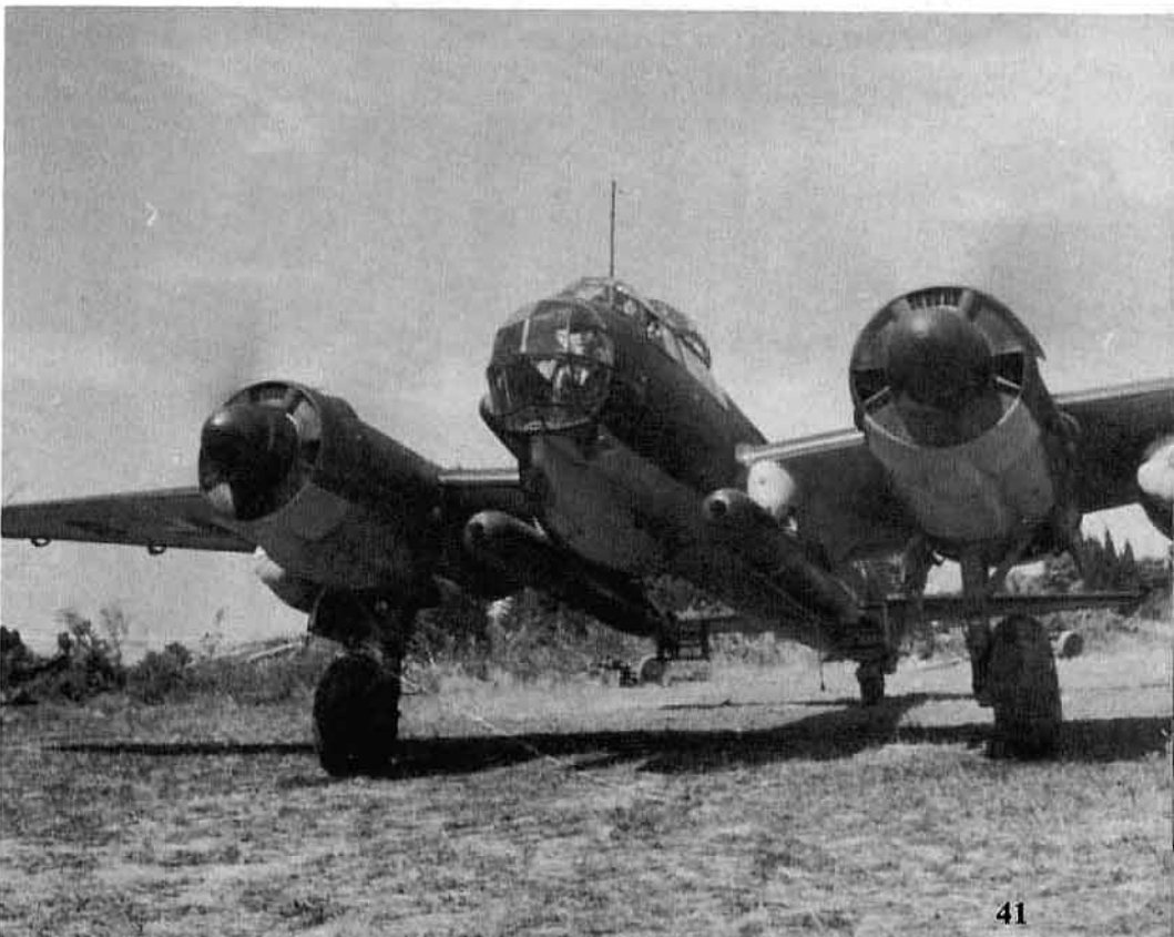
Carrying a pair of torpedos, a Ju 88A-4/Torp prepares for take-off with the aid of Walter rocket pods carried under each outboard wing. The bulged fairing for the torpedo control lines was on the starboard side of the nose only.
