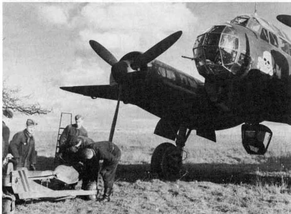
Luftwaffe armorers move a bomb loading cart under a Black bellied Ju 88A-1 of KG 54 Totenkopf (Death's head). The Ju 88 carries an optional MG 15 machine gun in the nose and has additional armor plate installed in the ventral gun position. The engine exhausts have been fitted with optional flame dampening shrouds.
