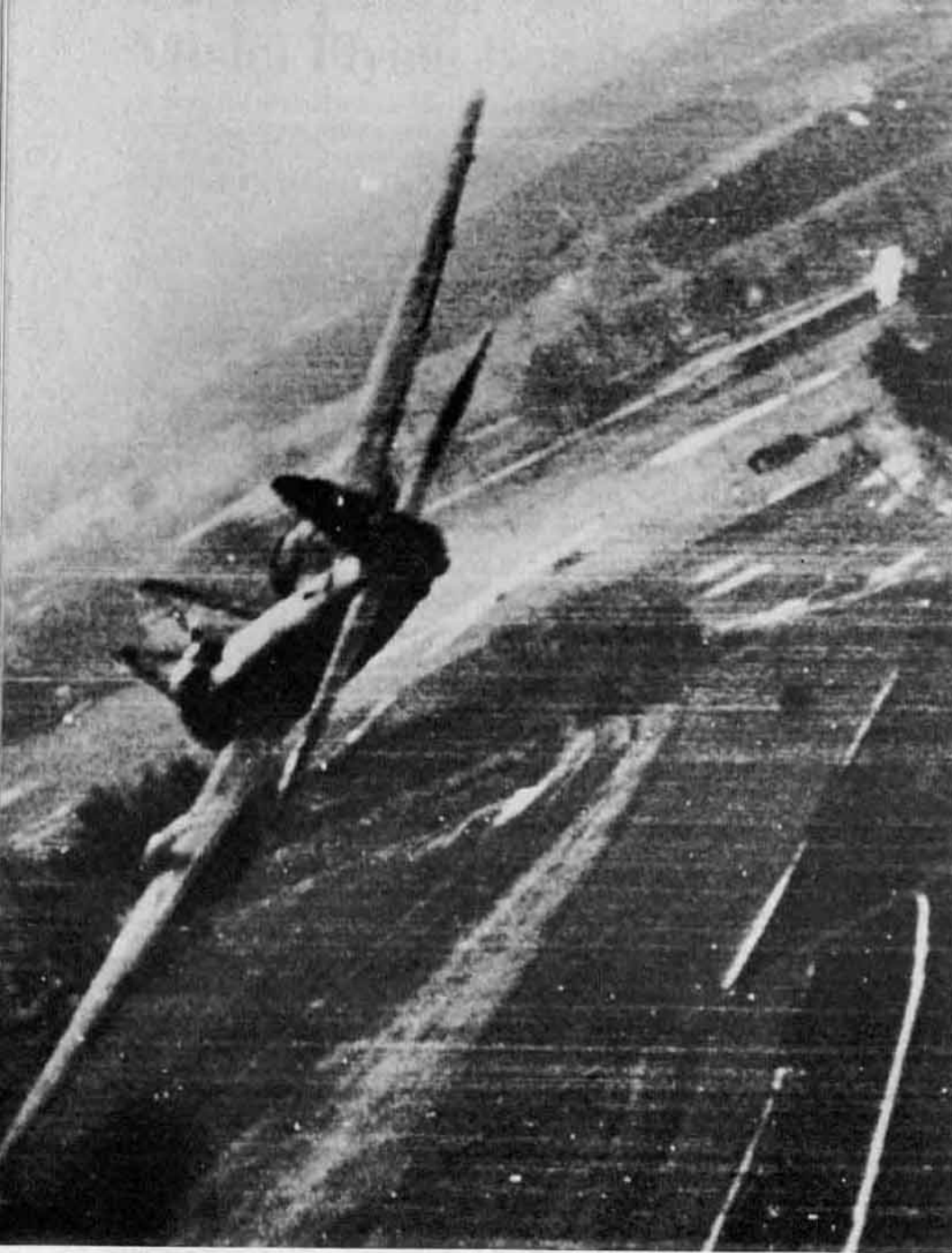
A Ju 88A-4 lower Mistel component was caught by USAAF P-51D Mustangs on 3 February 1945 and shot down. The drag of the fighter support structure and tail support catch yoke on the aft fuselage deck severely restricted the speed and maneuverability of the Ju 88 making it an easy kill!! (USAF)
