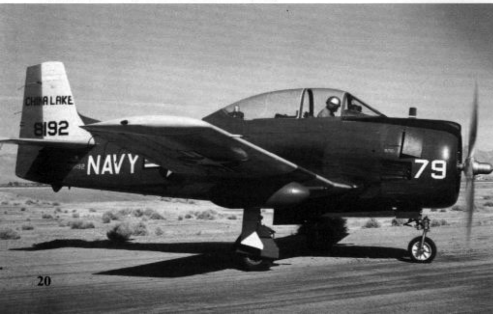
This T-28BD (BuNo 138192) was stationed at the Naval Weapons Test Center, NAF China Lake, California during May of 1958. The aircraft carries two underwing .50 caliber machine gun pods that enabled the Trojan to shot down the drone if control was lost and it threatened a populated area. (D.D. Olson via W.T. Larkins)
