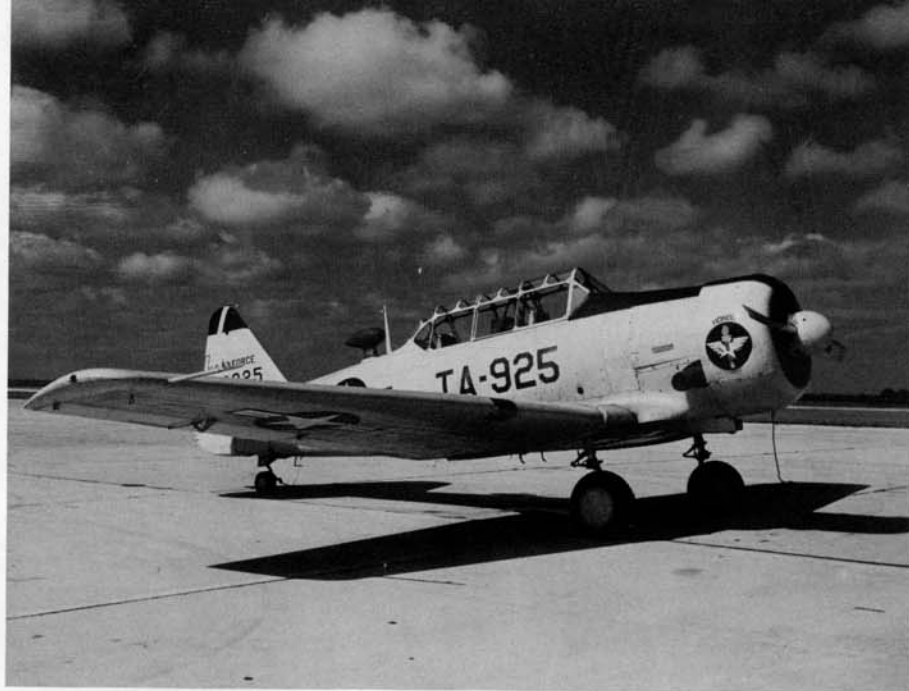
The commander of the training school at Hondo AFB used this T-6G as his personal aircraft. The tip of the tail is in Red, Yellow and Blue representing the squadrons under his command. The T-6G had a reduced frame canopy and a football shaped direction-finding (DF) antenna housing behind the cockpit. (Dorr)
