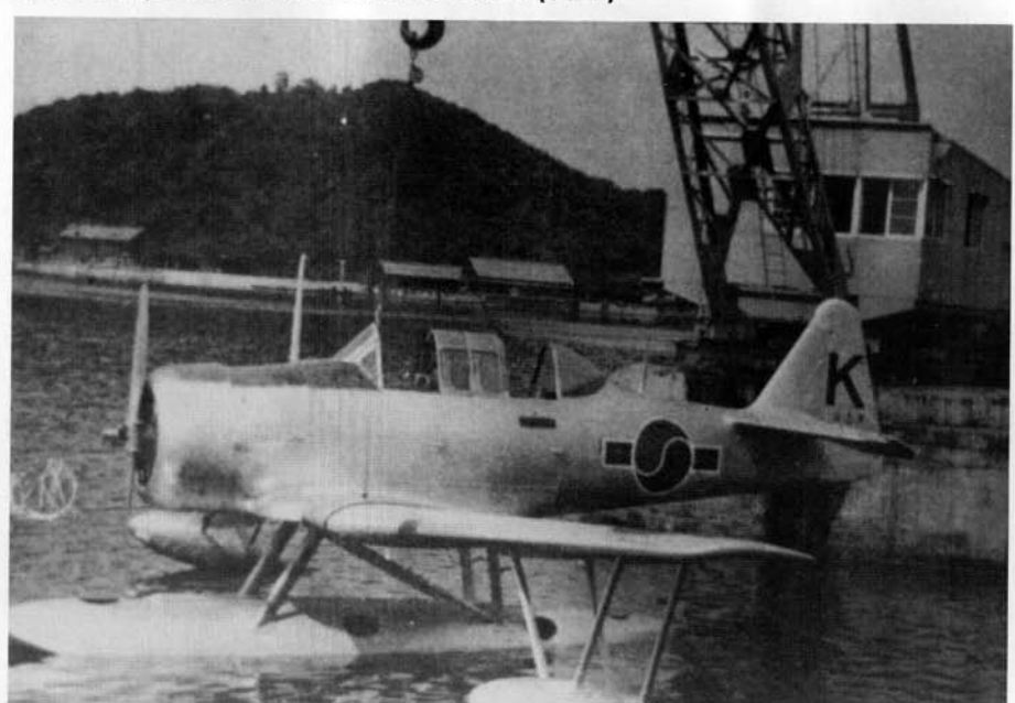
The ROK Navy's first aircraft was this T-6 floatplane. The 6147th T-6F ran out of gas and crash landed at Kwangju in December of 1950. ROK and US crews hauled the wreck to Chinhae where they modified it with the center float from a Japanese Rufe and wing tip floats made from F-80 tip tanks. It was known as the KN-1. (USAF)
