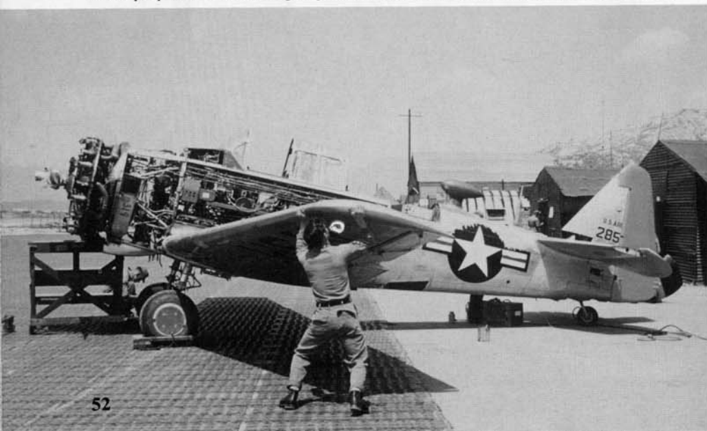
This AT-6D Texan of the 6147th TCS at K-47 during 1951 has been stripped of its fuselage skin in preparation for undergoing intermediate maintenance. (Mosquito Association)
