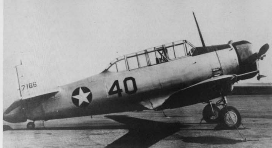
This BT-9B (37-166) has had the fabric-covered fuselage panels replaced with all-metal panels from a BT-14. The poor fit of the panel joint line under the tail is a result of the length difference between the BT-9 and BT-14 which made it necessary to trim the panels. (Taylor)
