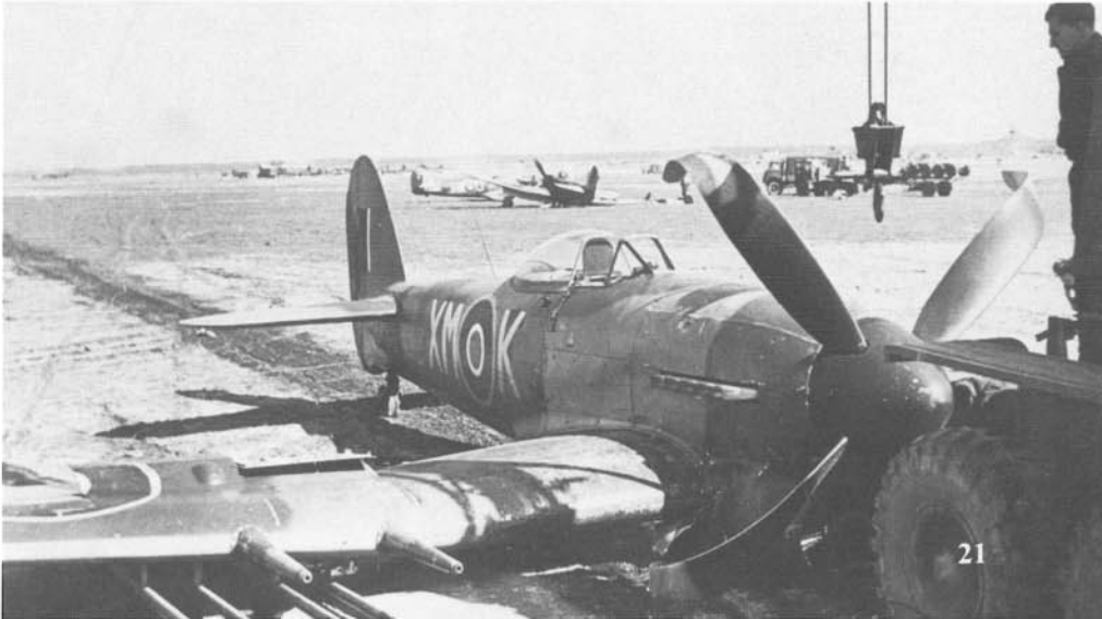
A salvage truck prepares to lift this Typhoon IB of No 182 Squadron back onto its landing gear after its pilot was forced to belly land the aircraft at Eindhoven on 24 March 1945.
