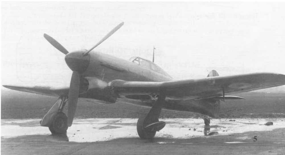
The second Typhoon prototype featured hinged wheel well doors on the landing gear legs, which were deleted on production aircraft in favor of separate doors. The prototype also had small windows mounted in the solid fairing behind the cockpit.
