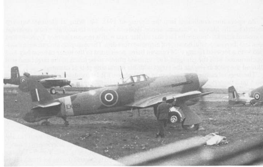
This Typhoon IB (EK128) suffered Category B damage on 30 January 1944 and was repaired during July by No 511 Forward Repair Unit. The aircraft was returned to service and saw action with Nos 174 and 137 Squadrons.
