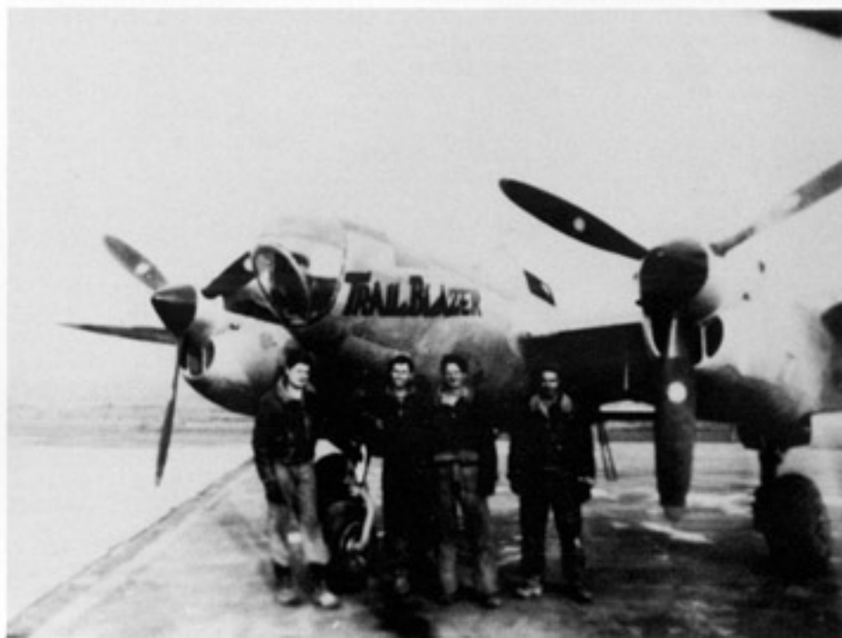
TRAIL BLAZER was a P-38J Droop Snoot of the 393th FS/367th FG based at Frankfurt, Germany during 1945. The Droop Snoot conversion included a Norden bombsight, bombing controls, additional oxygen and complete navigational equipment. (SGT James Crow)
