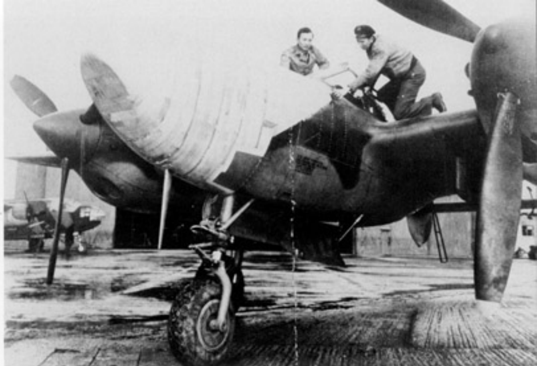
This P-38H (42-67086) was used to create and test the shape of the Droop Snoot bombardier nose for the P-38. The mockup nose was shaped from solid wood and was later used as a mold for the production Plexiglas nose. (AFM)
