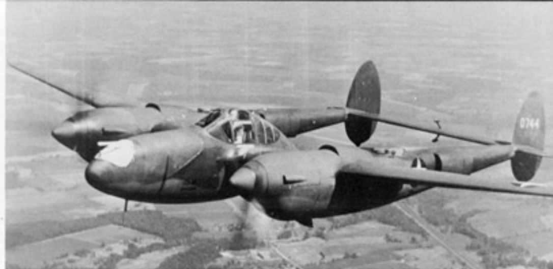
The first production P-38-LO (40-744) conducts a test flight over California during mid-1941. The P-38-LO was identical to the YP-38 except for the installation of armament and a more blunted tip on the propeller spinner. These aircraft were delivered in Olive Drab over Neutral Gray camouflage. (AFM)
