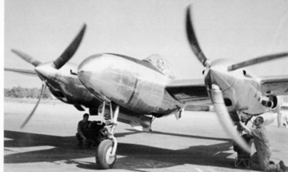
Lockheed Test Pilot Marshall Headie warms up the YP-38 on the Lockheed ramp prior to a test during September of 1940. The propellers on the YP-38 rotated in opposite directions — outward, toward each wingtip. (Lockheed)
