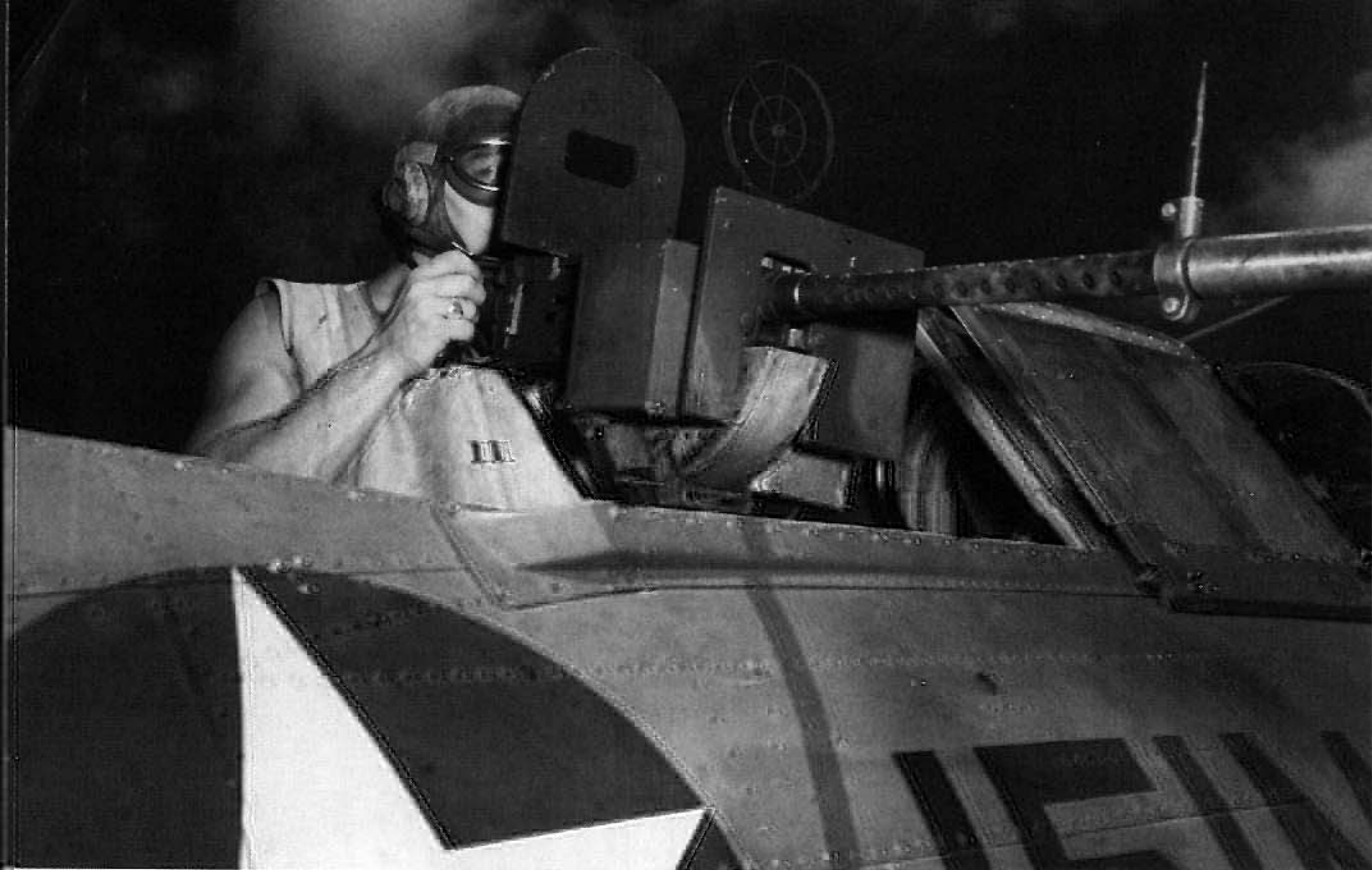
A Marine Corps enlisted radioman/gunner mans the air-cooled Browning .30 caliber machine gun in the rear cockpit of an SBC-4 on Santee during 1942. The gun has been modified with a ring and blast sight and an armor shield for the gunner. To use the gun, the rear fuselage turtledeck had to be folded down and the rear cockpit canopy was slid forward. This aircraft was SBC-4, which was named Miss Irene. (National Archives via R. J. Crossman)
