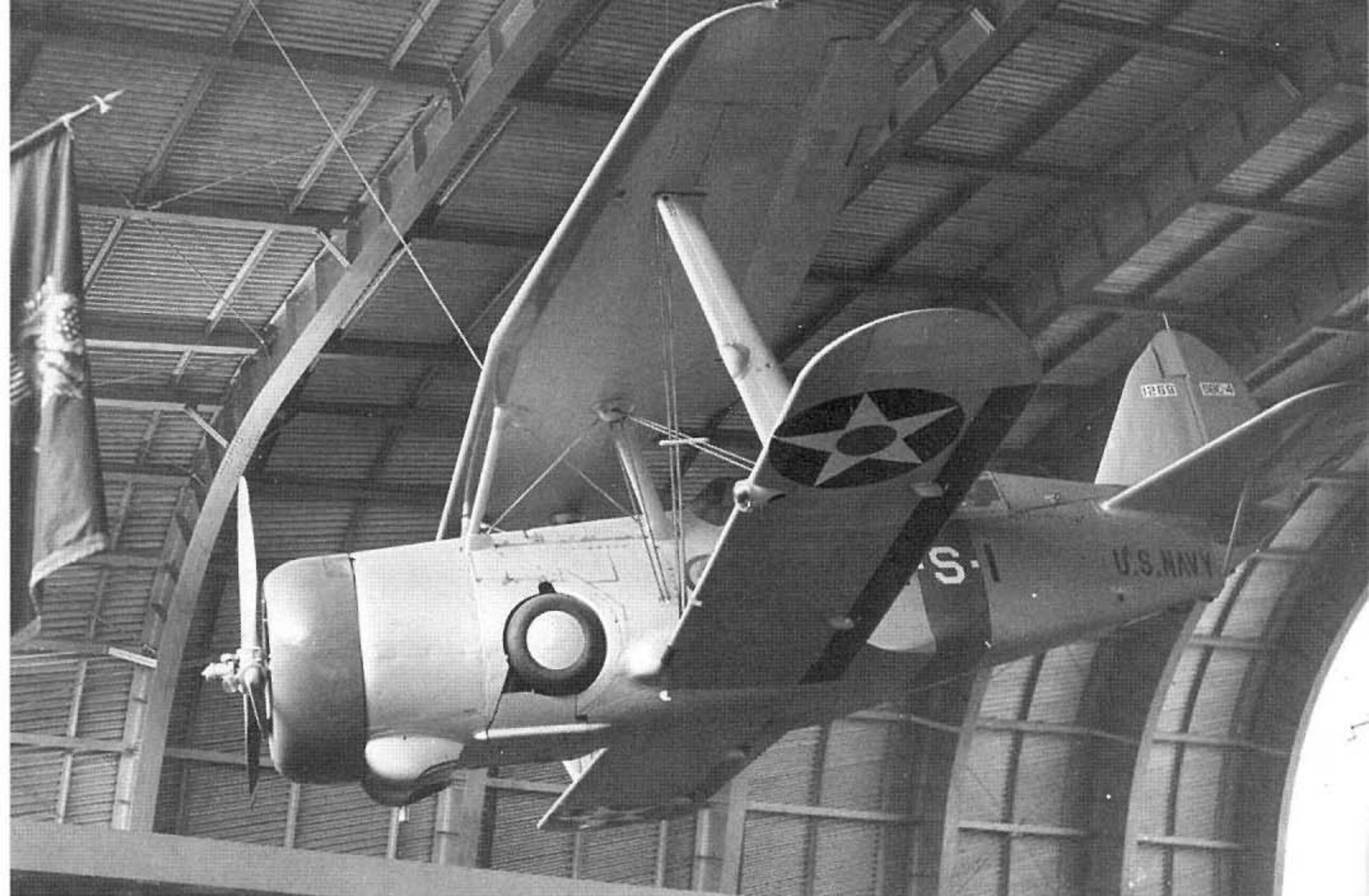
A SBC-4 (BuNo 1269) on display at the New York Worlds Fair of 1939. The aircraft had non-standard fairings over the exhaust stubs. The aircraft later served with VS-2 where it carried the side code 2-S-12 during October of 1940. (H. Clark via D.W. Lucabaugh)
