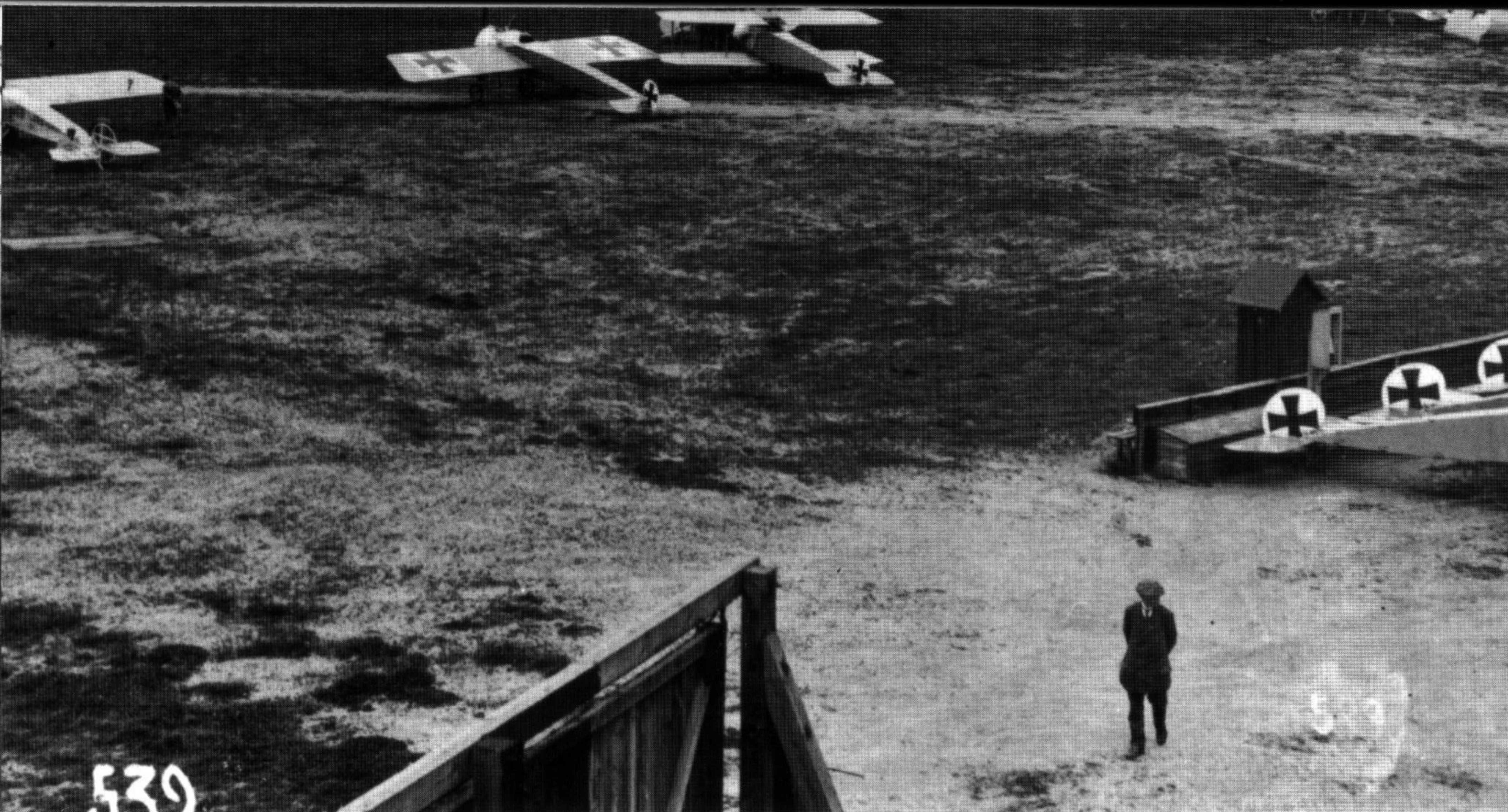
The air park at the Fokker factory in Schwerin. A number of Fokker M.14Vs (E.III) are parked just inside the fence and the aircraft on the grass include an E.III (left) covered in a clear cover intended to make the aircraft less visible. This technique was tested, but found to be of little value and was abandoned. (Fokker)
