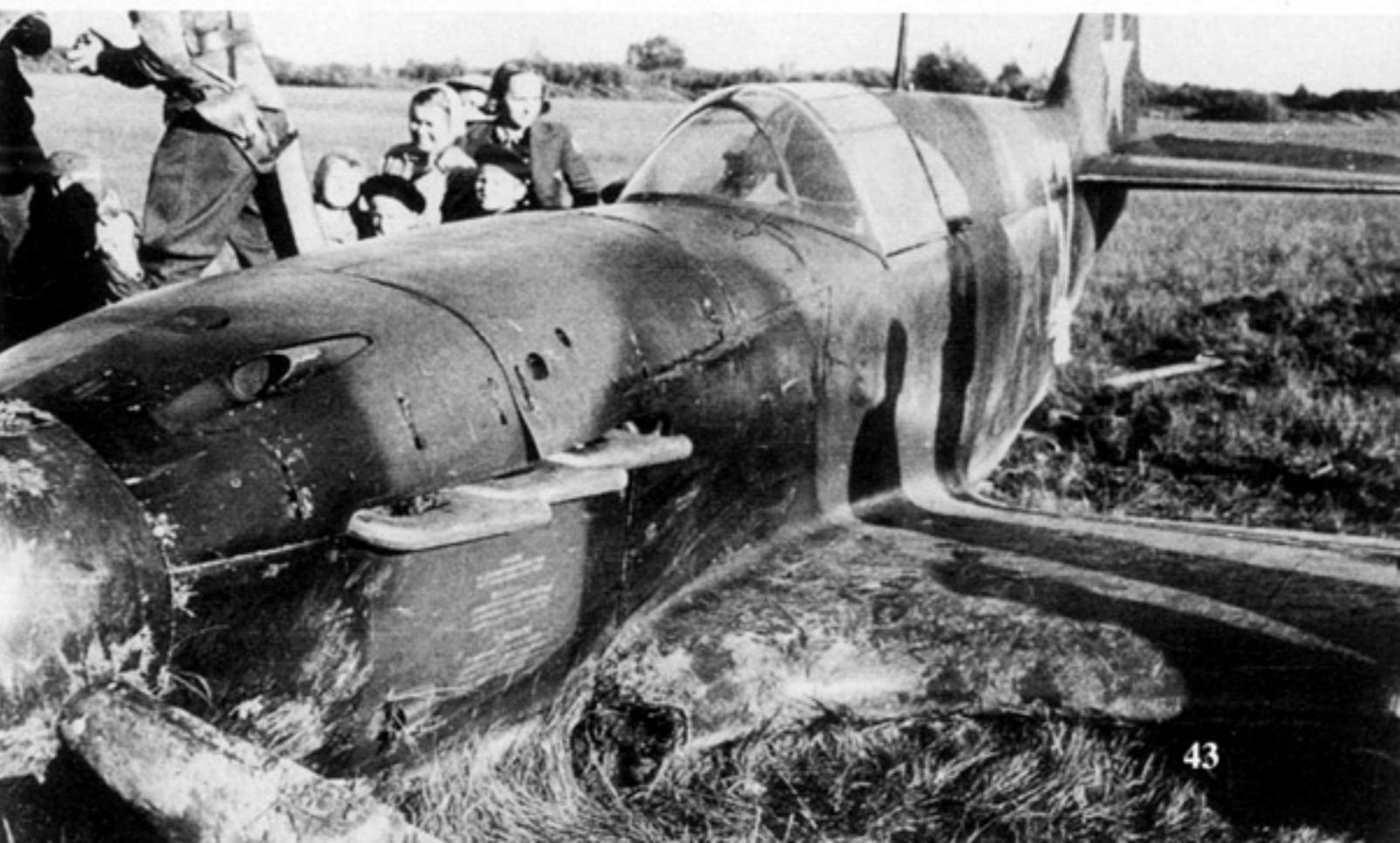
On 14 September 1942, Soviet and Finnish fighters clashed over the Finnish held Olonets Isthmus. One LaGG-3 (35th Series) was damaged by Alto Tervo and belly landed in a meadow at Ala-Sedoksa, where it drew considerably attention from the local habitants. The muzzle for the Berezin UBS 12.7MM machine gun is clearly visible. (Keski-Suomen Ilmailumuseo via Hannu Valtonen)
