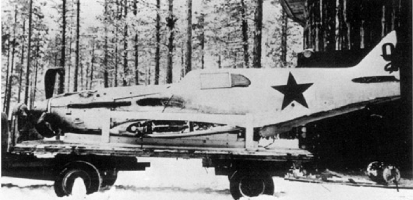
Red 29, a LaGG-3 (4th Series) was captured by the Finnish Air Force at Aunus during early 1942. It was transported by truck to a repair depot for rebuilding. The tactical number had been applied to the tail over the national marking. (Keski-Suomen Ilmailumuseo via Hannu Valtonen)
