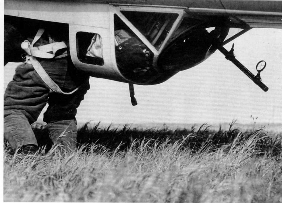
The ventral gunner enters the He 111P's gondola prior to a mission over Poland in 1939. One 7.92MM MG 15 was fitted to the aft window, allowing for protection of the bomber's rear and lower areas. The weapon is fitted with a post-and-ring gunsight, with the post near the breech and the ring near the muzzle. (Bundesarchiv)
