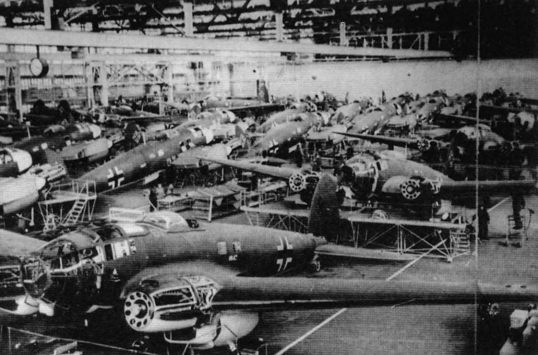
Several He 111Ps approach the final assembly section at a German factory in 1939. Other aircraft move in the opposite direction to be mated with the wing assemblies later in the production line. Production of the Jumo 211-powered He 111H began concurrently with the He 111P, although at different factories. (Werkfoto via Petrick)
