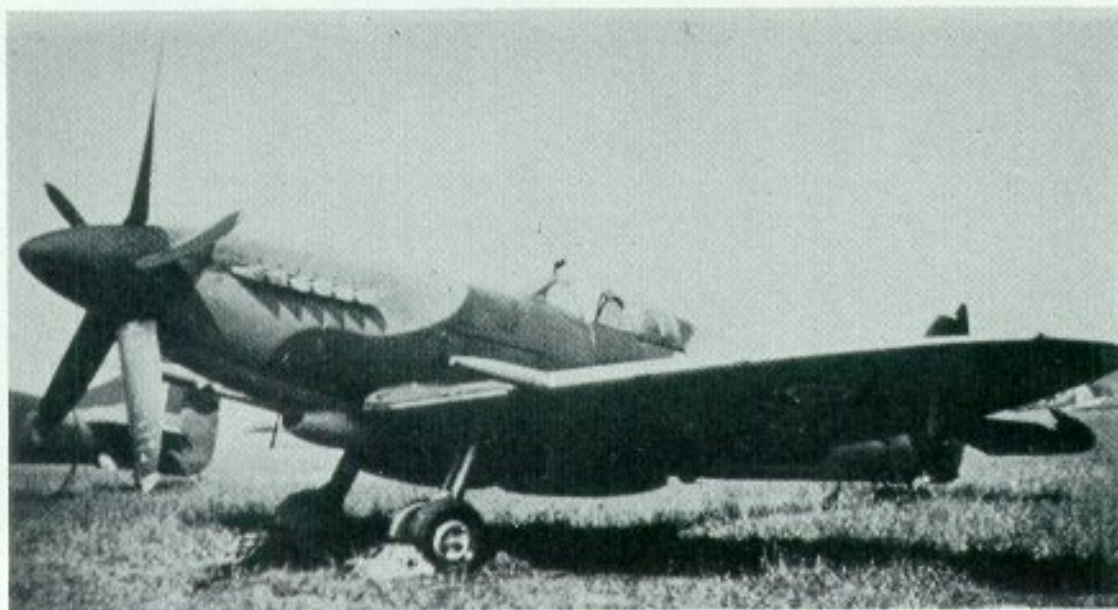
Production Spitfire F.Mk.XIV C (RB159), coded DW-D of No. 610 Squadron, Auxiliary Air Force, RAF, shows off the two big radiators and long-range drop tank. (Photo: IWM, CH.13811)
