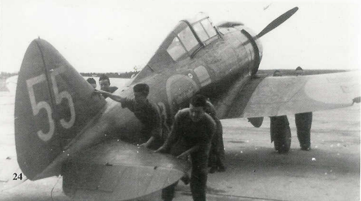
RSAF ground crewmen check the tail of a J-9 at Barkarby during the Summer of 1941. Several J-9s were modified for the reconnaissance mission with a pair of aerial cameras mounted behind the pilot in the fuselage spine. To aid in rapid identification, the wing insignia was greatly oversized. (AFM)
