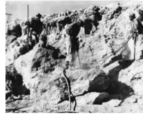
Chilean miners drill for nitrates with jackhammers.
