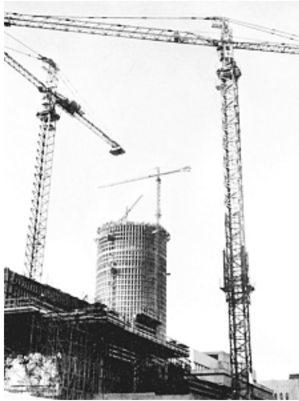
Figure 3-27 Tower crane on a building site. (Courtesy of Potain Tower Cranes, Inc.)
