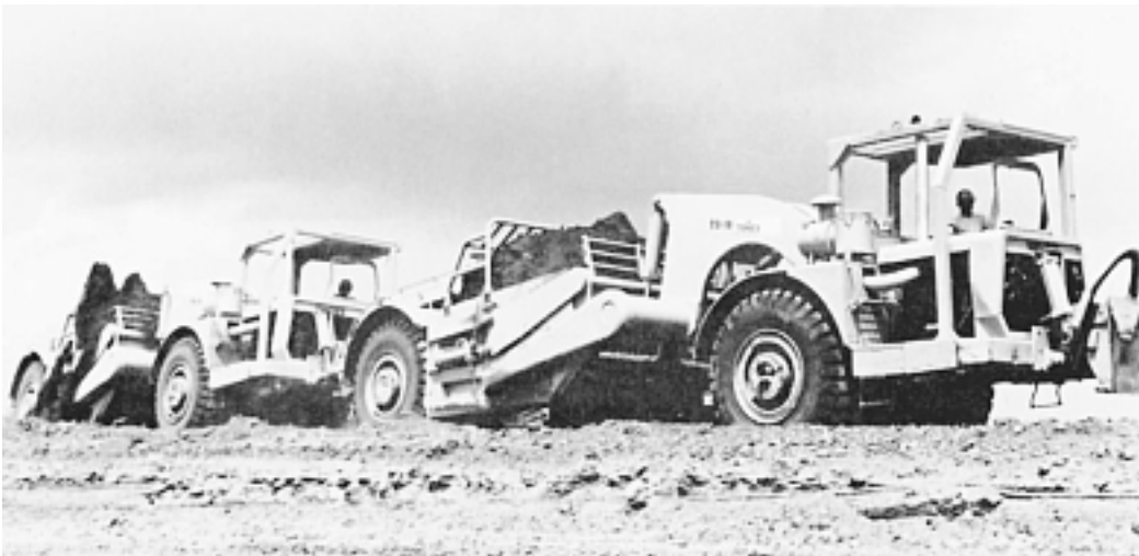
Figure 4-19 Twin-hitch scraper loading. (Courtesy of CMI Terex Corporation)
