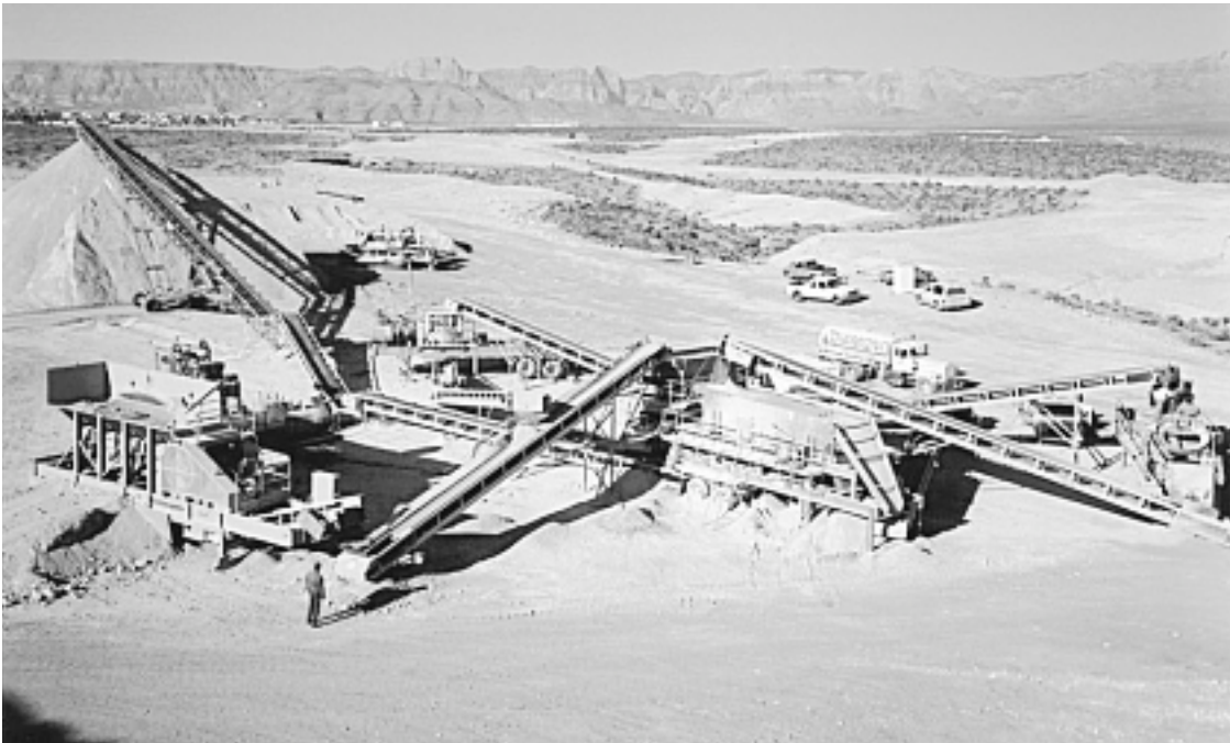
Figure 7-1 Aggregate processing plant. (Courtesy of Cedarapids, Inc.)
