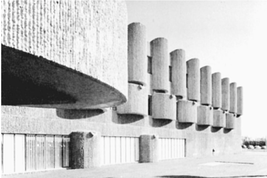
Figure 12-14 Mechanically produced concrete surface texture. (Courtesy of Portland Cement Association)
