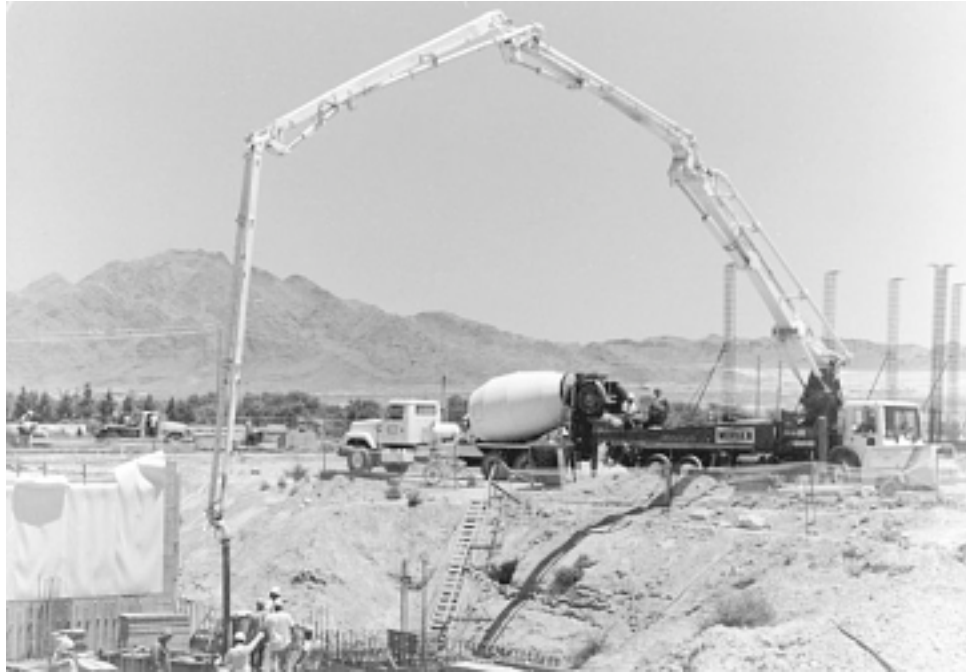
Figure 12-15 Concrete pump and truck mixer. (Courtesy of Morgen Manufacturing Co.)
