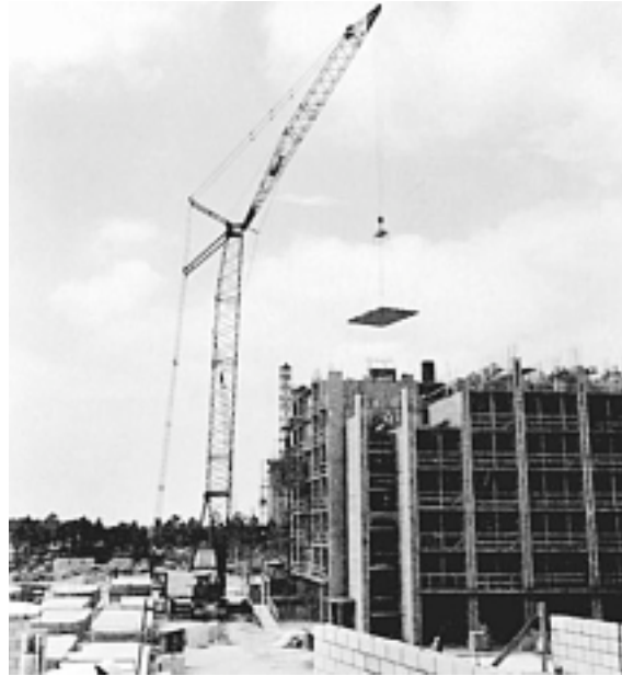
Figure 12-26 Repositioning flying form. (Courtesy of CMI Terex Corporation)
