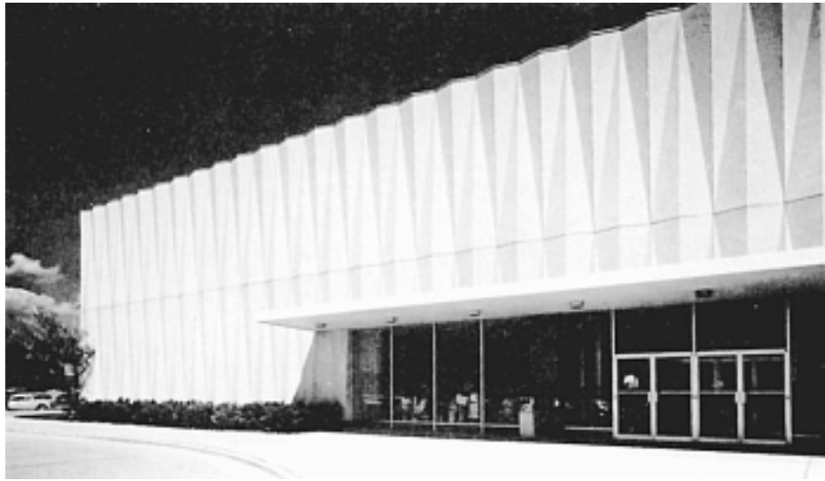
Figure 12-12 Application of architectural concrete. (Courtesy of Portland Cement Association)
