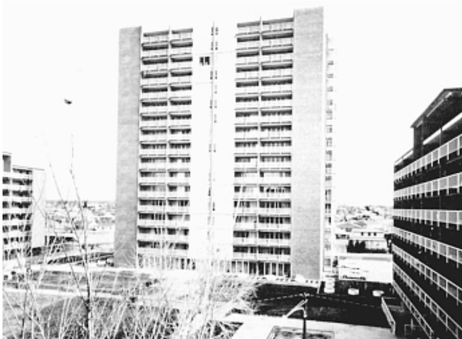
Figure 14-10 Seventeen-story building constructed with reinforced brick masonry bearing walls. (Courtesy of The Brick Industry Association)
