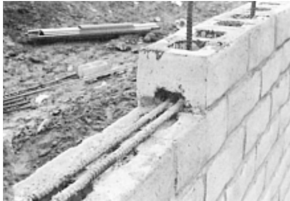
Figure 14-17 Construction of a high-rise motel using reinforced concrete masonry walls. (Courtesy of Portland Cement Association)
