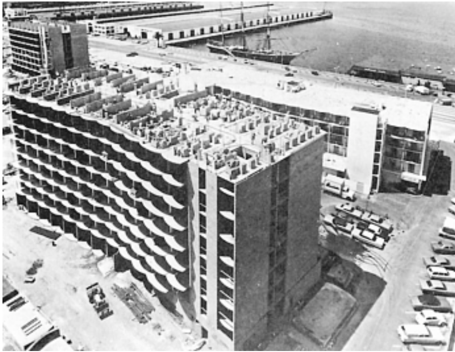
Figure 14-17 Construction of a high-rise motel using reinforced concrete masonry walls. (Courtesy of Portland Cement Association)
