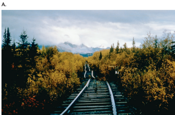
FIGURE 15.21 A. When a rail line was built across this permafrost landscape in Alaska, the ground subsided. (Photo by Lynn A. Yehle, U.S. Geological Survey) B. In places in Alaska, a pipeline is suspended above ground to prevent melting of delicate permafrost. (Tom & Pat Lesson/Photo Researchers)
