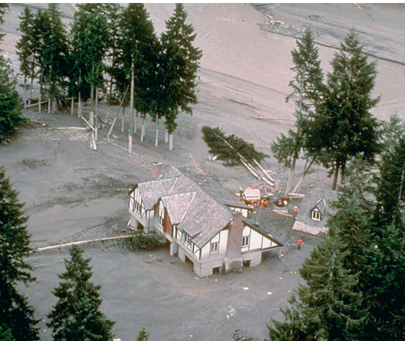
FIGURE 15.15 A house damaged by a lahar along the Toutle River, west-northwest of Mount St. Helens. The end section of the house was torn free and lodged against trees. (Photo by D. R. Crandell, U.S. Geological Survey)
