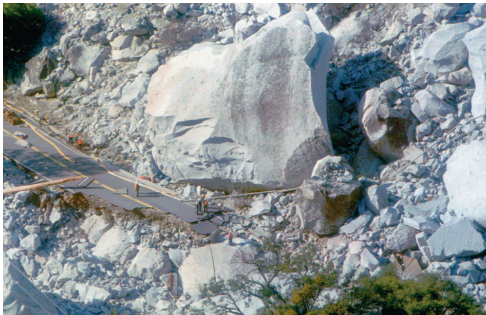
FIGURE 15.9 In January 1997, this rockfall blocked Highway 140 near the Arch Rock entrance to Yosemite National Park, California. (Photo by Roger J. Wyan/AP/Wide World Photos)
