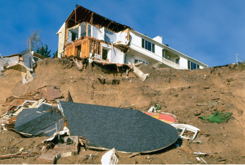
FIGURE 15.7 Various forms of mass wasting can be triggered by earthquakes. This home in Pacific Palisades, California, was destroyed by a landslide triggered by the January 1994 Northridge earthquake. In some cases, damages from earthquake-induced mass wasting are greater than damages caused directly by an earthquake's ground vibrations. (Photo by Chromo Sohm/Corbis/The Stock Market)
