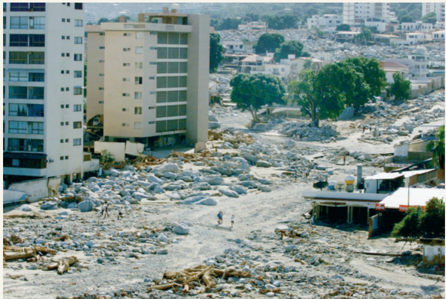
FIGURE 15.G Debris-flow damage. Huge boulders (in excess of 300 tons) were transported by some flows. (AP/Wide World Photo)
