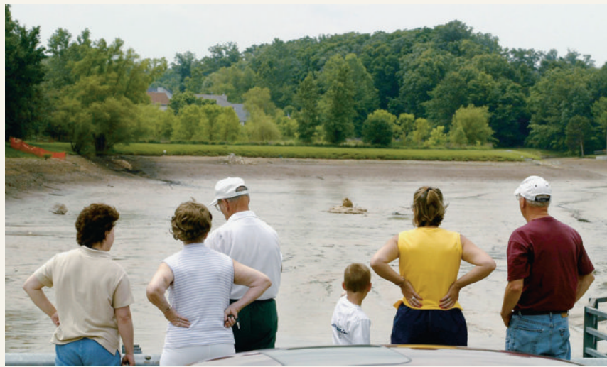
FIGURE 17.D Residents examine emptied Lake Chesterfield, a 23-acre reservoir that drained in three days when a sinkhole opened beneath it. (Photo by Hillary Levin/ St. Louis Post Dispatch )
