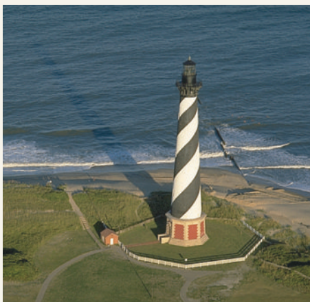
FIGURE 20.A When North Carolina's historic Cape Hatteras Lighthouse was threatened by coastal erosion, it was moved in the summer of 1999. Here you see the lighthouse before it was moved when it was only about 100 meters (330 feet) from the water. (Photo by Don Smetzer/Getty Images Inc.—Stone Allstock)
