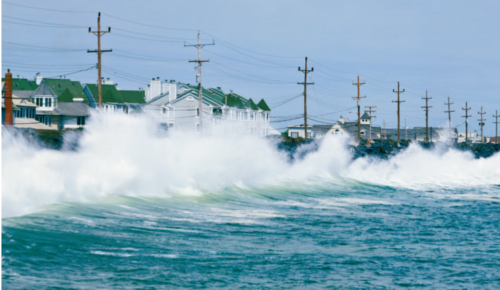
FIGURE 20.20 Seabright in northern New Jersey once had a broad, sandy beach. A seawall 5 to 6 meters (16 to 20 feet) high and 8 kilometers (5 miles) long was built to protect the town and the railroad that brought tourists to the beach. As you can see, after the wall was built, the beach narrowed dramatically. (Photo by Rafael Macia/Photo Researchers, Inc.)
