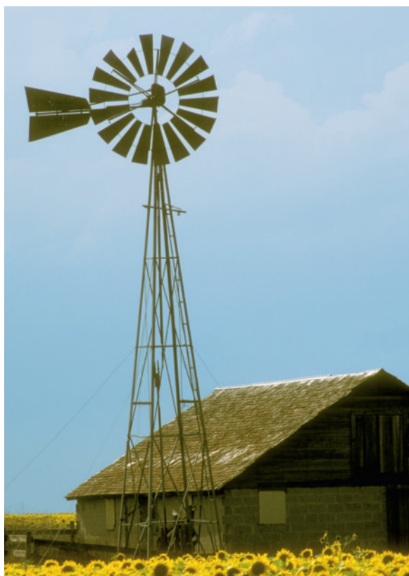
FIGURE 23.13 A. Farm windmills are still familiar sights in some areas. Mechanical energy from wind is commonly used to pump water. (Photo by Darren Bennett) B. The use of wind turbines for generating electricity is growing rapidly. These turbines are at Crowley Ridge, Alberta, Canada. (Photo by Alan Sirulnikoff/Photo Researchers, Inc.)
