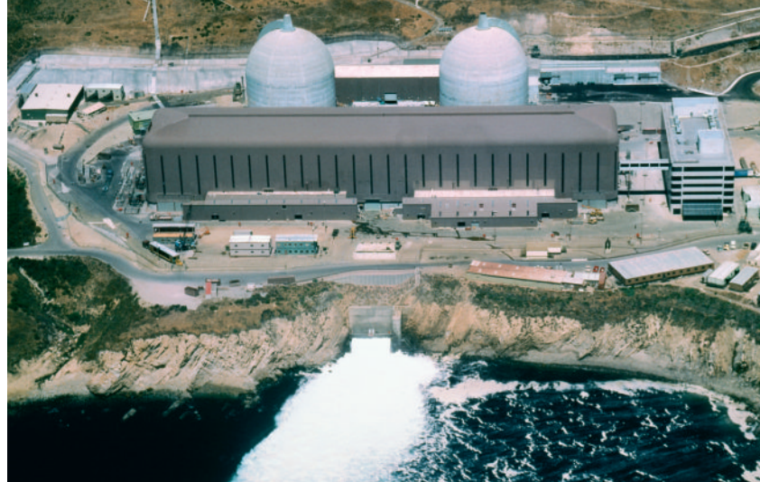
FIGURE 23.11 Diablo Canyon nuclear power plant near San Luis Obispo, California. Reactors are in the dome-shaped buildings, and cooling water is being released to the ocean. The setting of this facility was controversial because of its close proximity to faults capable of producing potentially damaging earthquakes. (Photo by Comstock)
