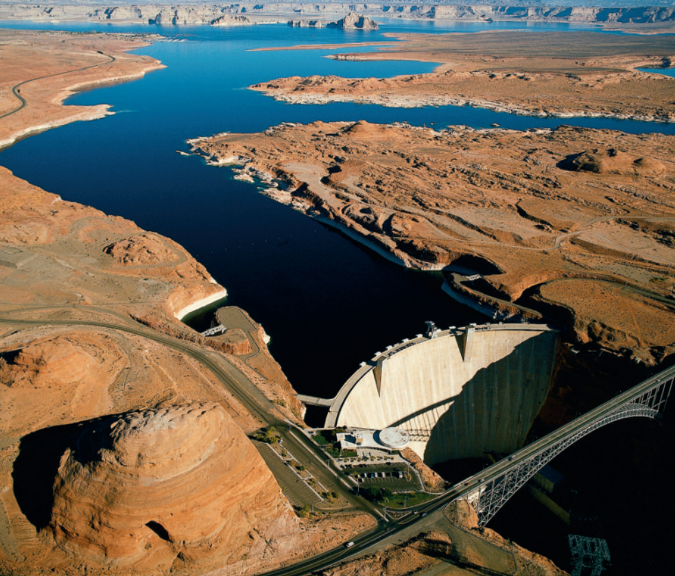
FIGURE 23.15 Lake Powell is the reservoir that was created when Glen Canyon Dam was built across the Colorado River. As water in the reservoir is released, it drives turbines and produces electricity. Eventually the reservoir will be filled with sediment deposited by the Colorado River. (Photo by Michael Collier)
