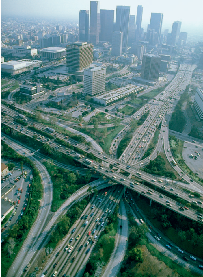
FIGURE 23.27 Crushed stone and sand and gravel are primarily used for aggregate in the construction industry, especially in cement concrete for residential and commercial buildings, bridges, and airports, and as cement concrete or bituminous concrete (asphalt) for highway construction. A large percentage is used without a binder as road base, for road surfacing, and as railroad ballast. (Photo by Robert Ginn/PhotoEdit)
