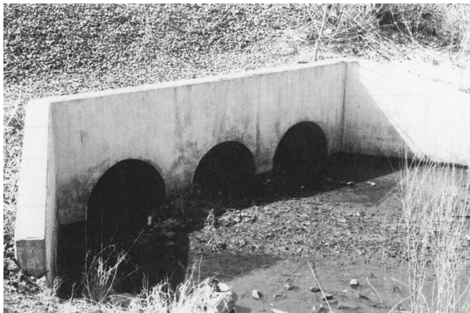
FIGURE 13-2 Typical three-barrel pipe culvert.
