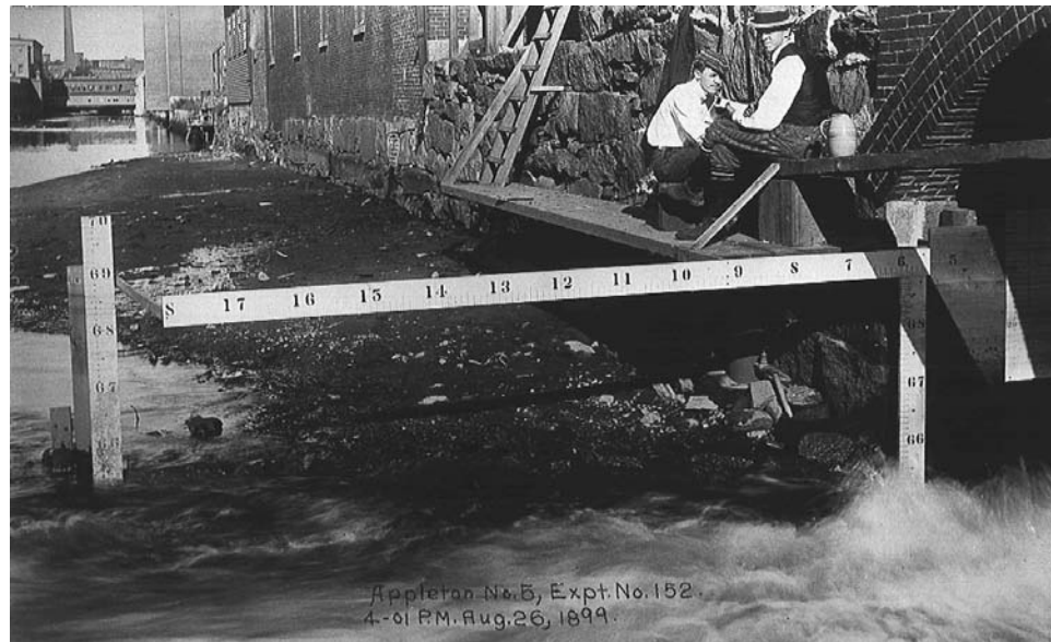
FIGURE 1-2 The city of Lowell, Massachusetts, was the site of a famous series of water power experiments conducted by James Francis and Uriah Boyden. The publication of the results in 1855 contributed greatly to the field of hydraulic engineering. Here, two assistants are shown measuring water levels. (Courtesy of University of Massachusetts Lowell, Locks and Canal Collection.)
