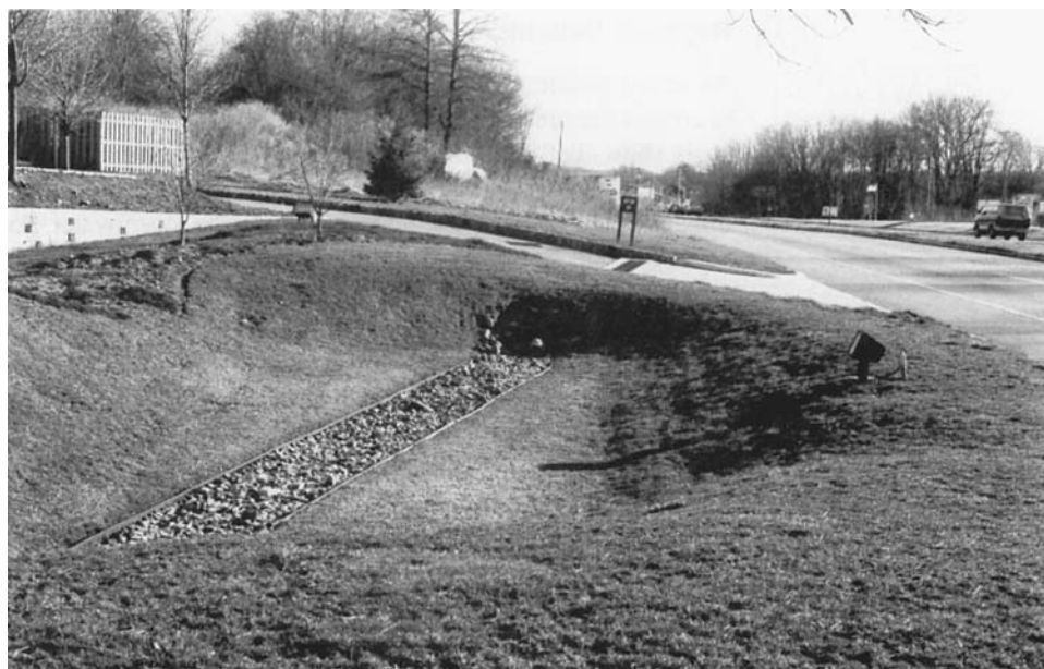
FIGURE 15-2 Typical small on-site detention basin. A riprap low-flow channel runs down the center of the basin.
