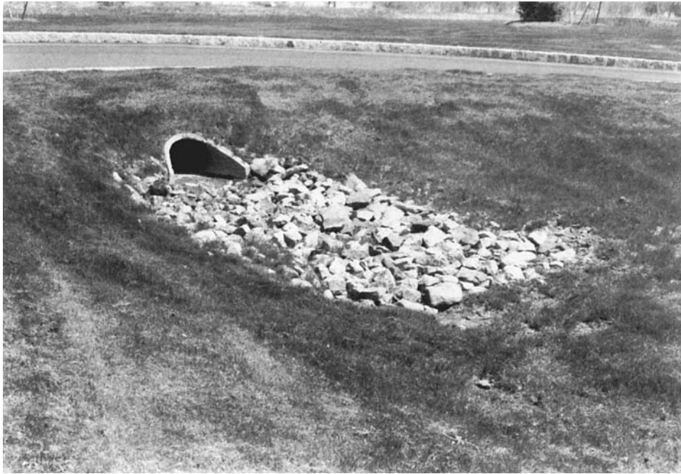
FIGURE 12-16 Storm sewer outfall with riprap erosion protection in place.
