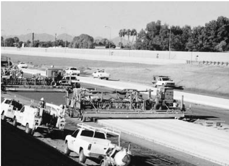
FIGURE 7.26 Curing concrete by machine applying membrane forming compound.
