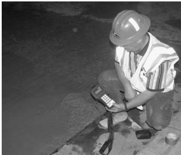
FIGURE 7.37 Checking the maturity of fresh concrete using the maturity meter.
