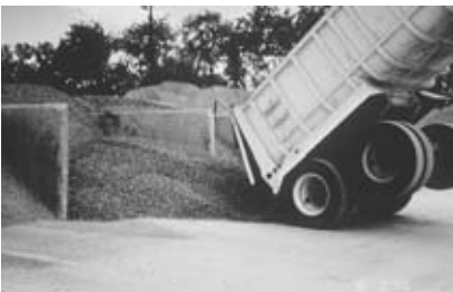
FIGURE 5.16 Aggregate bins used to stockpile aggregates with different sizes.
