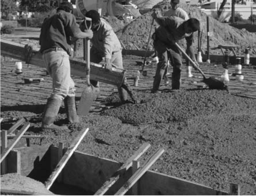
FIGURE 7.7 Pouring concrete slab.
