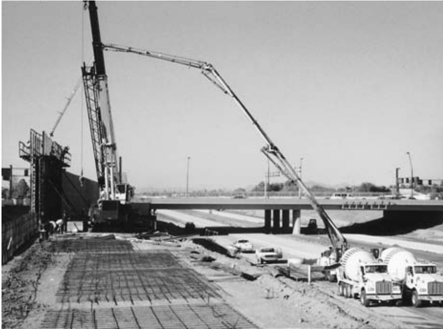
FIGURE 7.10 Pumping concrete in a retaining wall.
