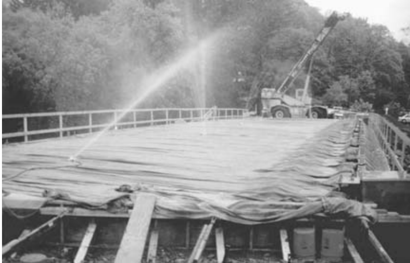
FIGURE 7.22 Curing concrete by wet covering.
