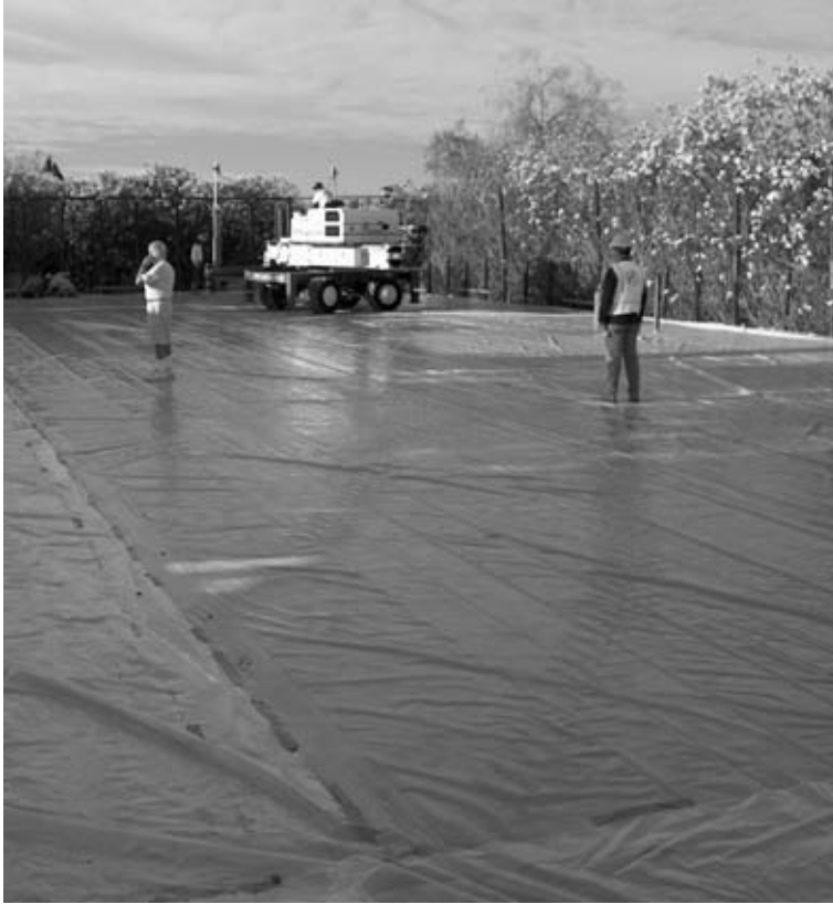
FIGURE 7.24 Curing concrete with plastic sheets.
