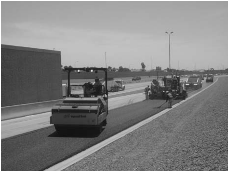
FIGURE 9.4 Compaction of hot mix asphalt.
