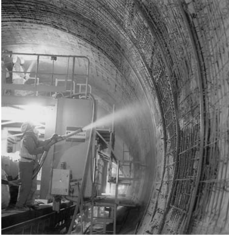
FIGURE 7.41 Shotcrete used in lining a tunnel.
