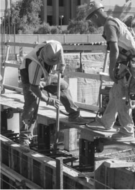
FIGURE 7.11 Consolidating concrete with an internal vibrator.
