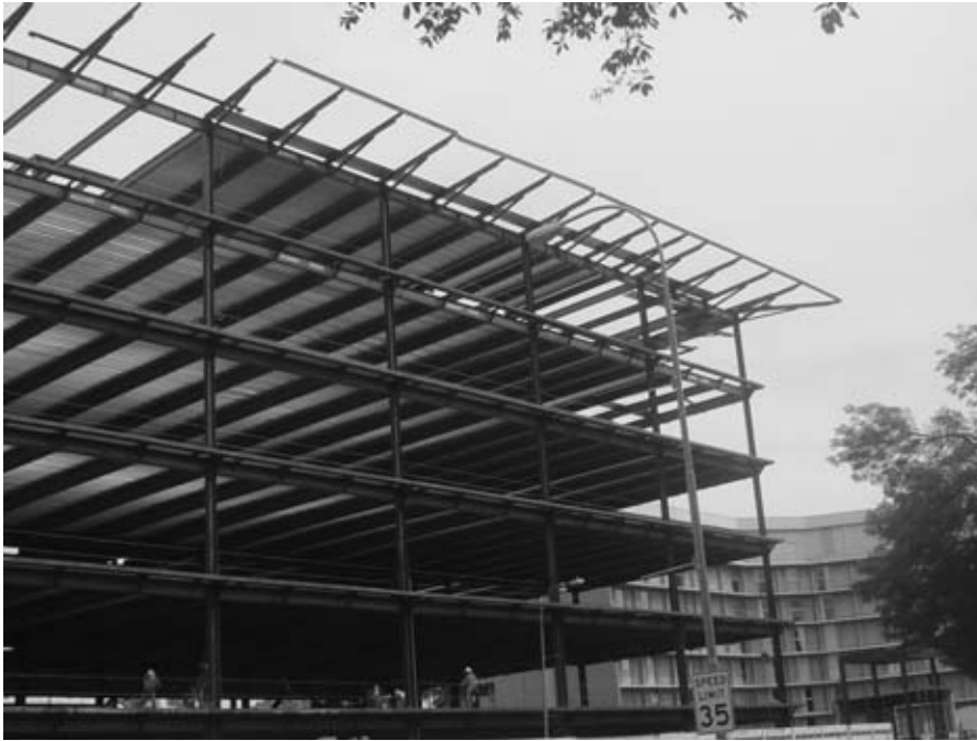
FIGURE 3.8 Structural steel used to make columns, beams, and floors for the structural support of a building.
