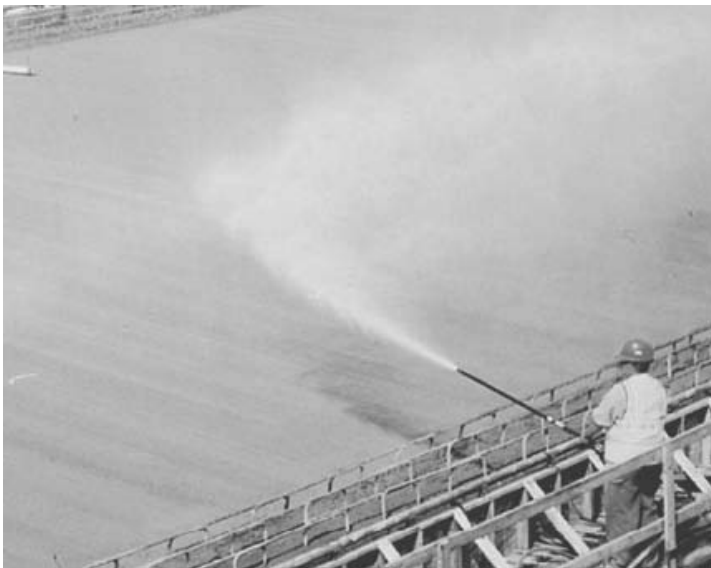
FIGURE 7.21 Curing concrete by fogging.
