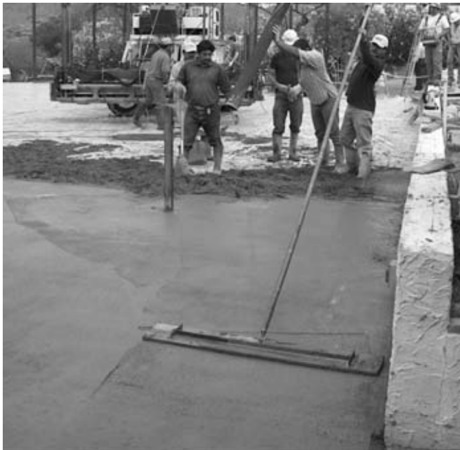
FIGURE 7.16 Finishing concrete with a straightedge.
