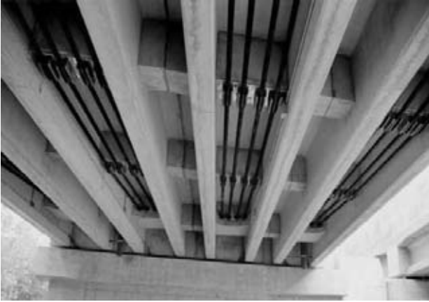
FIGURE 11.9 Strengthening a concrete bridge with FRP bars.
