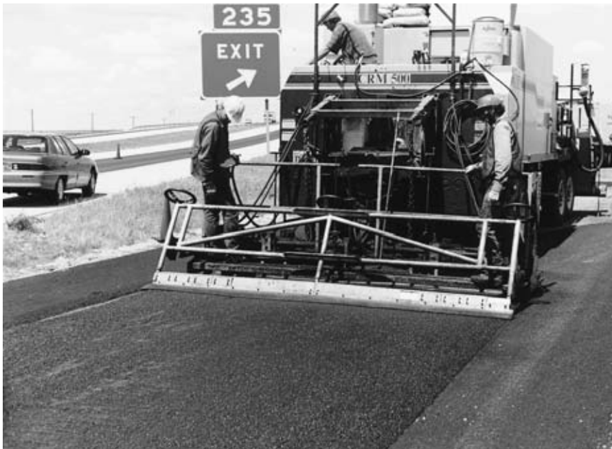
FIGURE 9.6 Applying microsurfacing for preserving existing pavement.
