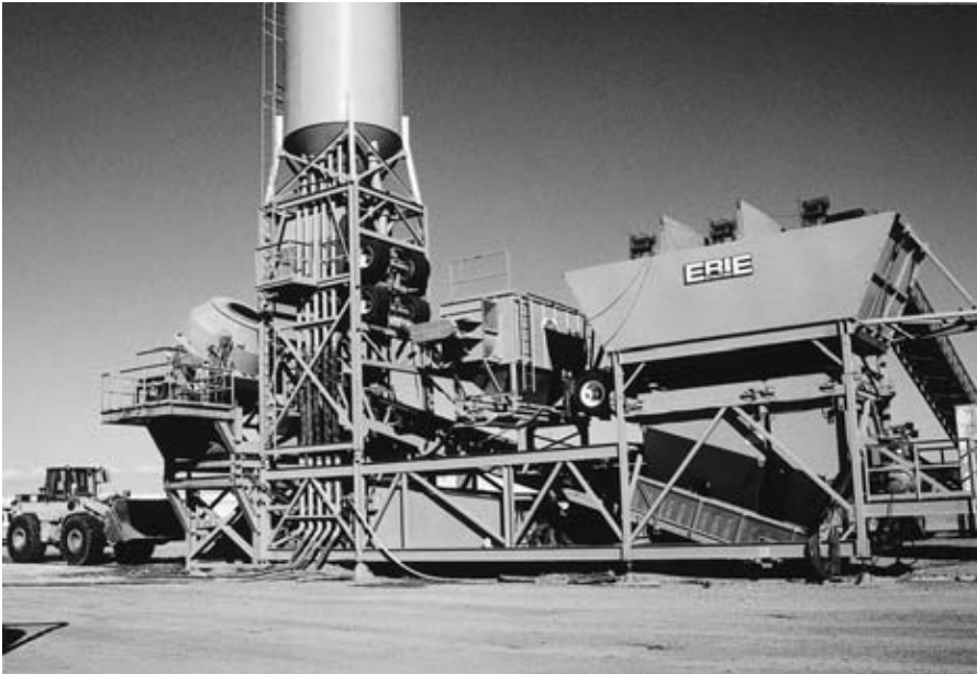
FIGURE 7.5 Mobile batcher mixer at the job site.
