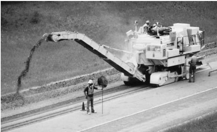
FIGURE 9.39 Milling old pavement.
