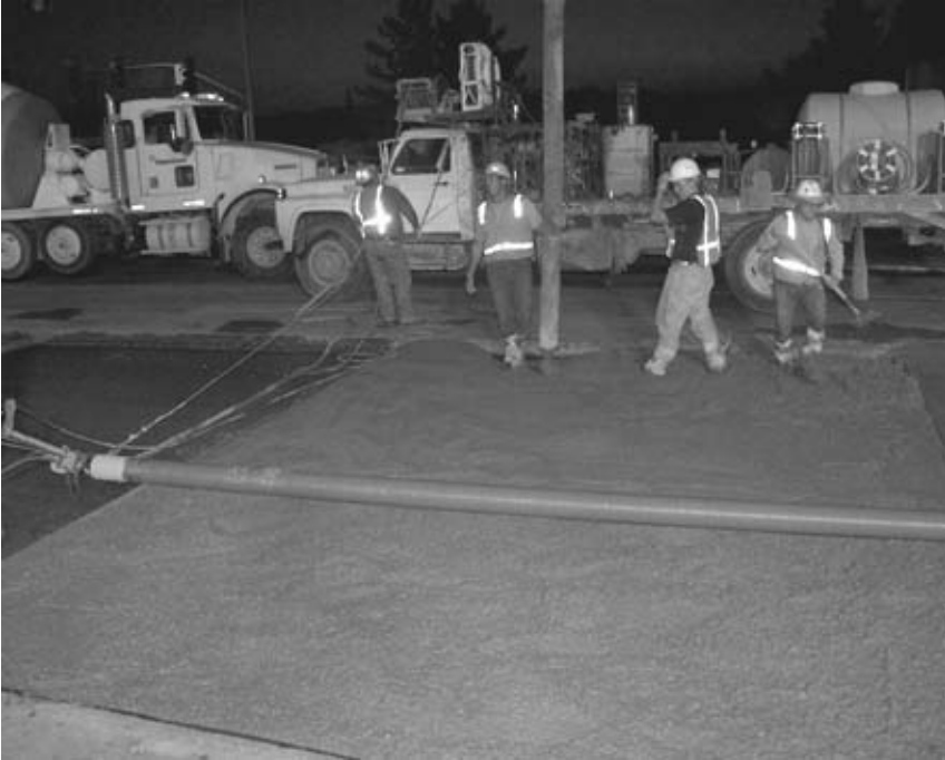
FIGURE 7.15 Spreading concrete with a straightedge.
