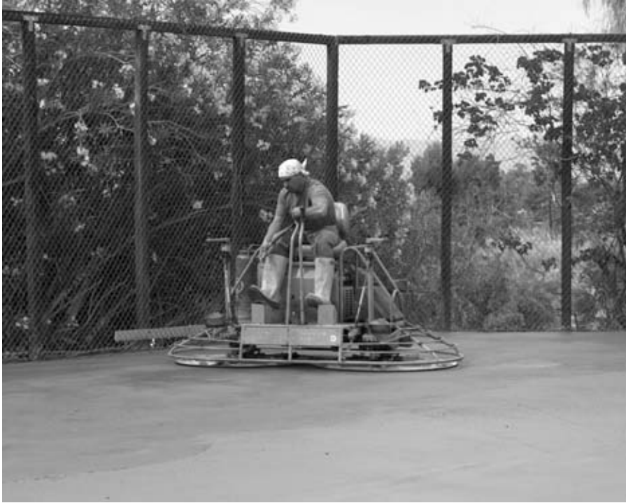
FIGURE 7.17 Finishing concrete with a power float.
