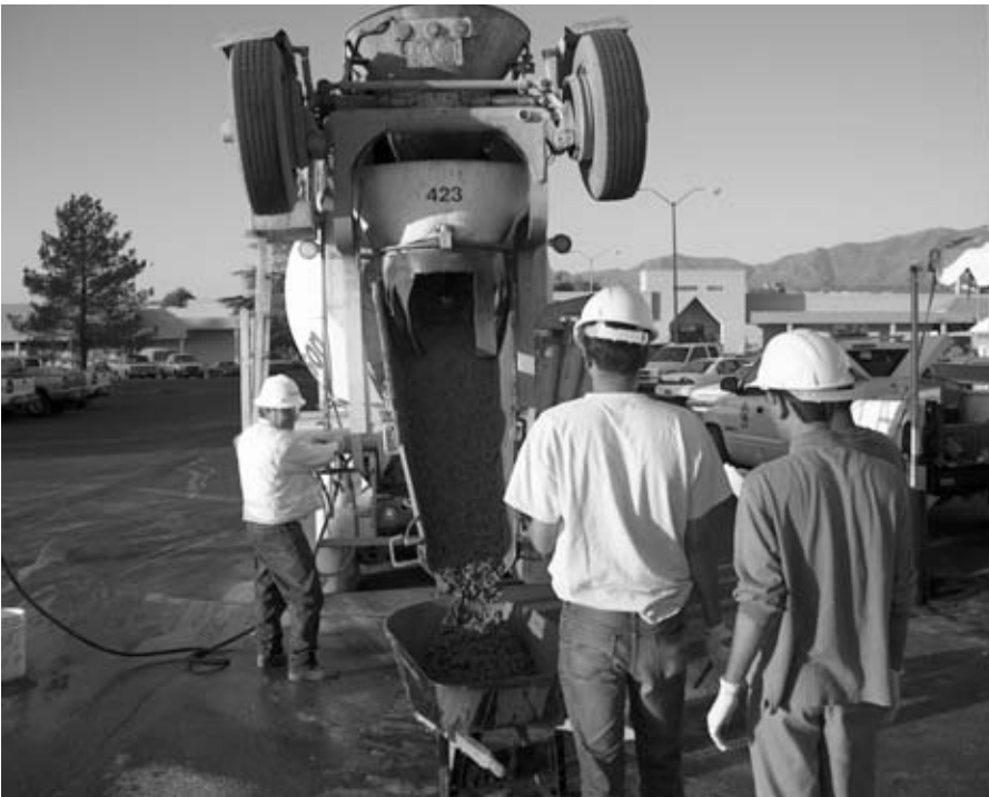
FIGURE 7.6 Loading concrete in a wheelbarrow.
