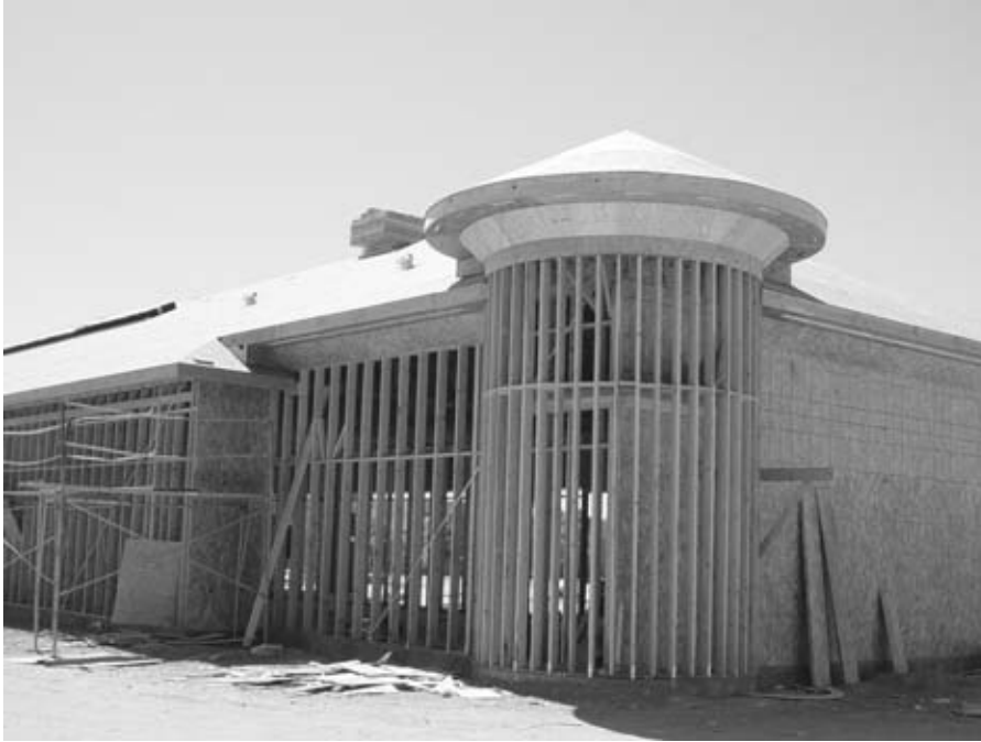
FIGURE 10.1 Wood frame used for building structural support.
