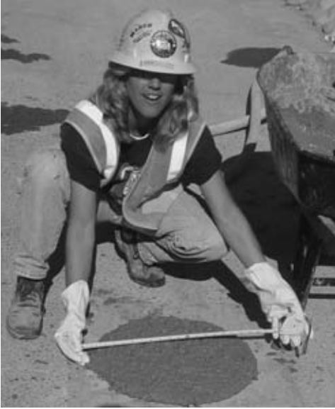
FIGURE 7.38 Measuring the spread during the slump flow test.
