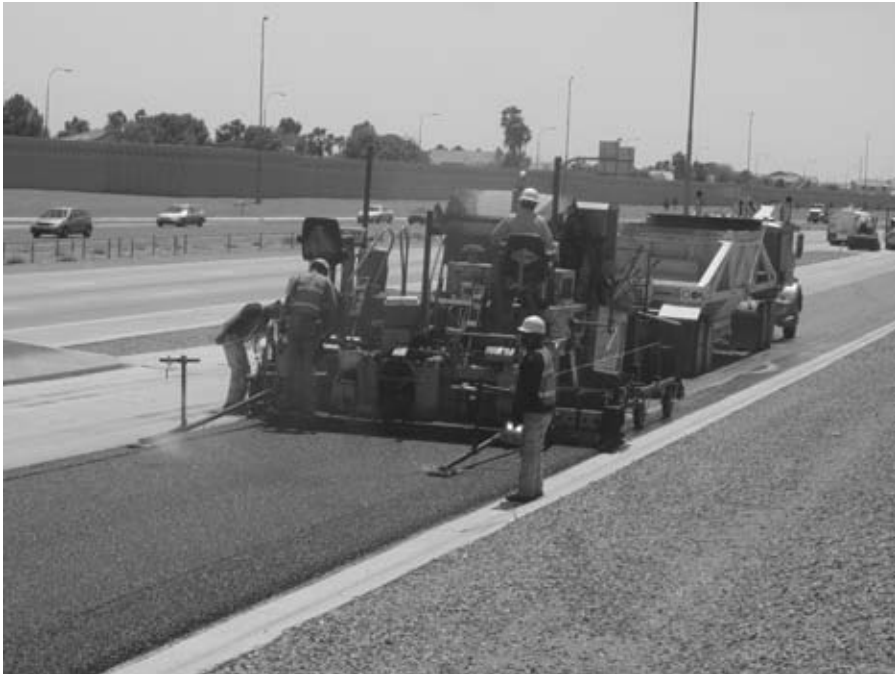
FIGURE 9.3 Placing hot mix asphalt (asphalt concrete) used for the surface layer of asphalt pavement.
