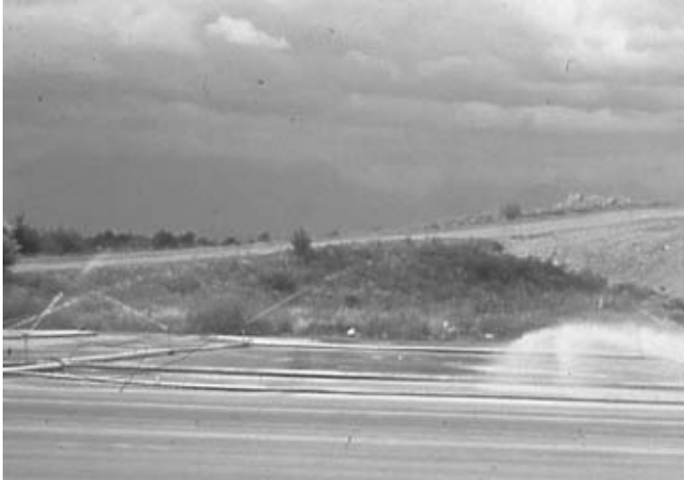
FIGURE 7.20 Curing concrete by spraying.
