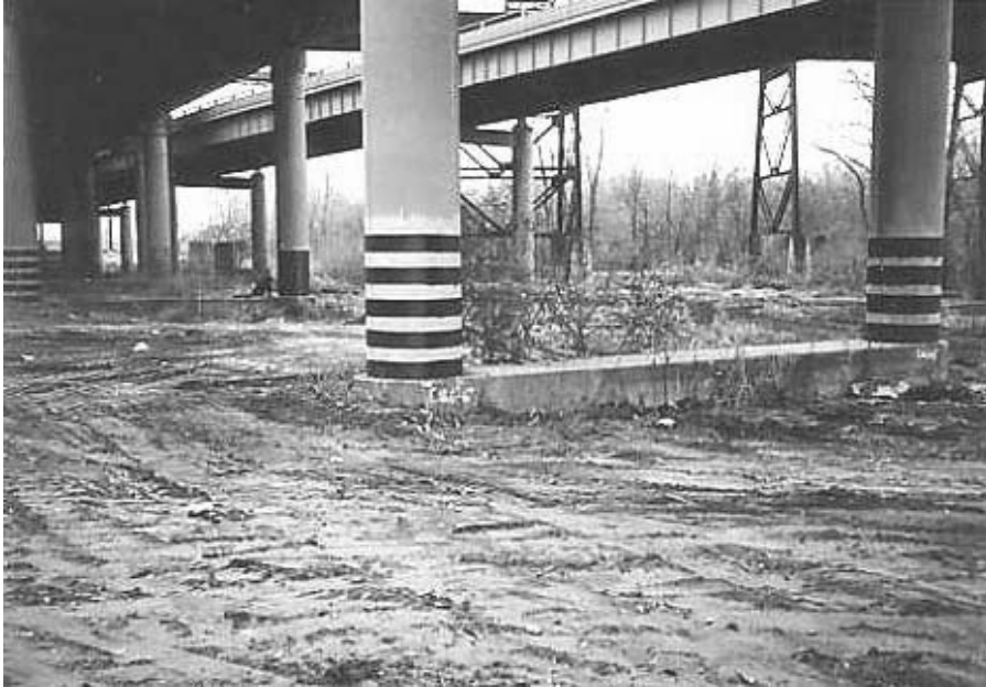
FIGURE 11.7 Wrapping columns of a bridge with FRP composites.
