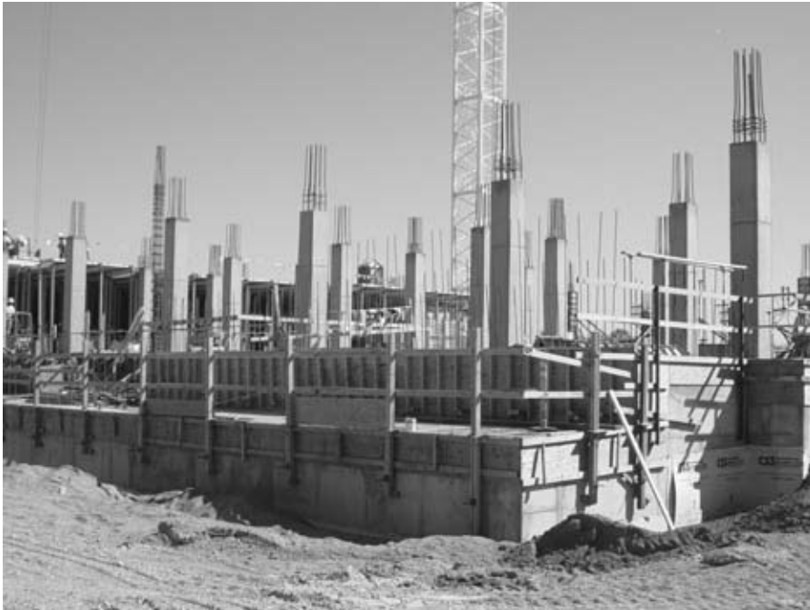
FIGURE 3.10 Steel rebar used to reinforce PCC columns.
