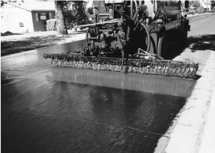
FIGURE 9.5 Applying fog seal for preserving existing pavement.
