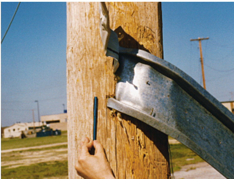
FIGURE 10-24 The force of the wind during a tornado near Wichita, Kansas, in April 1991 was enough to drive this piece of metal into a utility pole. (Photo by John Sokich/NOAA)
