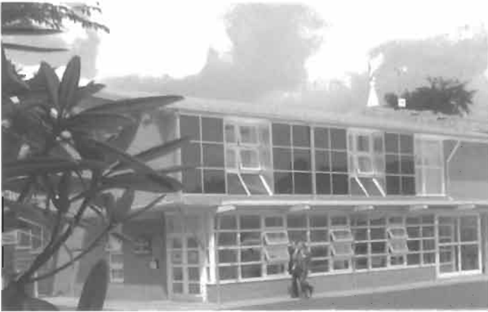
Figure 11 The facade panels used at the first floor level of this building in the Department of the Built Environment at Nottingham University each incorporate about 1 m 2 of thin film solar cells, but look almost identical to standard glazing panels.
