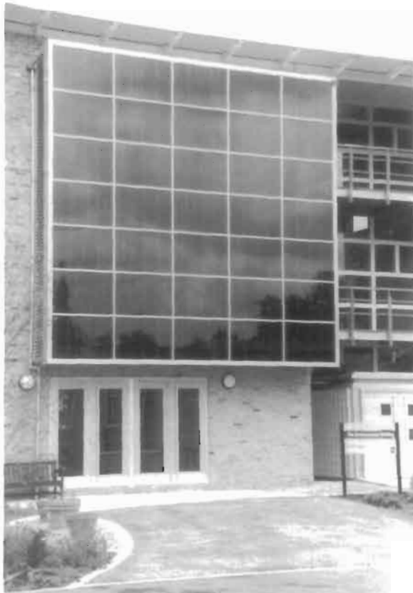
Figure 10 Office of the Future PV facade, Building Research Establishment, UK.
