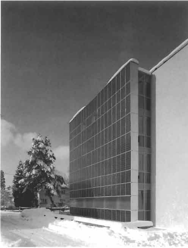
Figure 6 PV facade at Sonnepark Dornbirn, Austria. Source: IEA Task VII PV Database. © stromaufwärts. Reprinted with permission.
