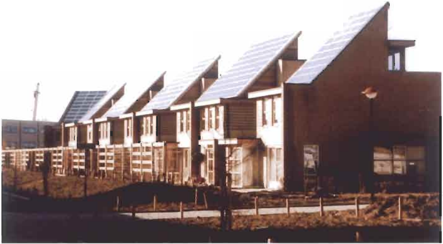
Figure 5 Sloped PV roofs at Amersfoort.
