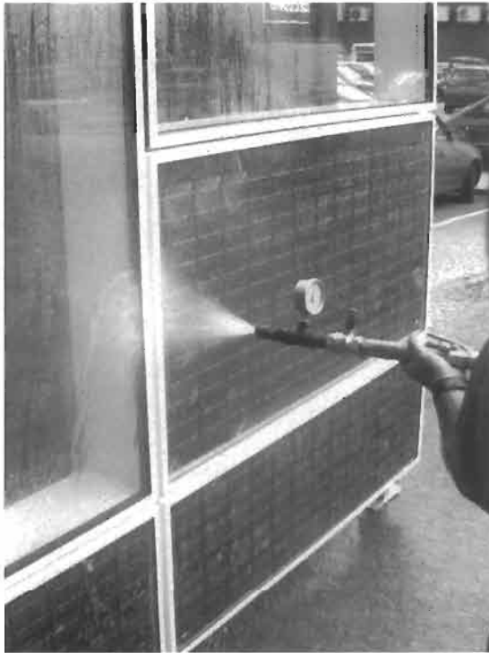
Figure 11 Pluswall PV facade, UK.
