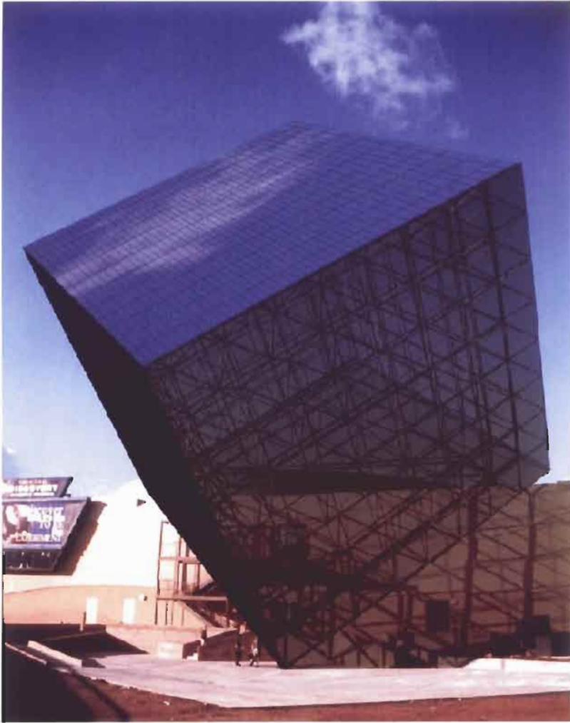
Figure 7 An independent PV structure: the giant solar cube in southern California. Photo courtesy of Steven Strong, Solar Design Associates, Harvard, MA, USA.
