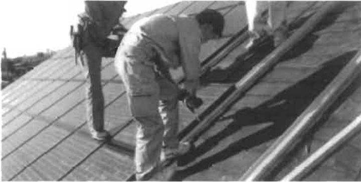
Figure 10 Installing a sloped PV roof. Source: IEA Task VII PV Database. © MSK Corporation. Reprinted with permission.
