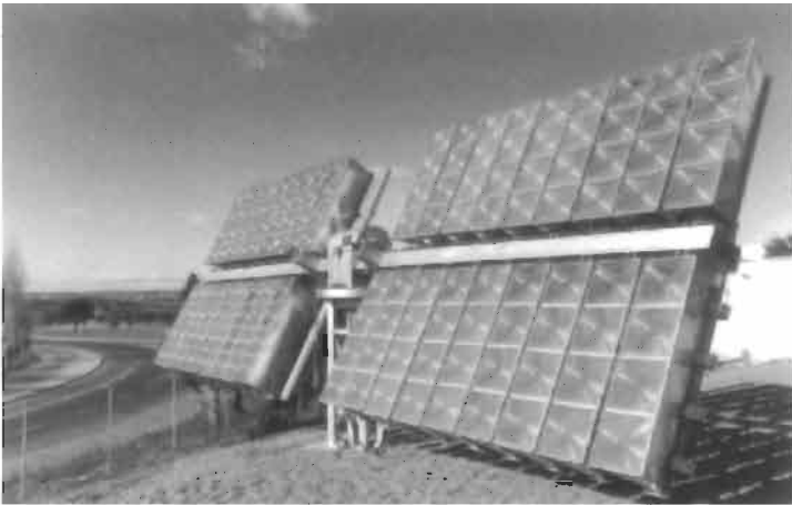
Figure 1 The Ramón Areces array (Madrid, 1980). One of the first 2 axis tracking European PV concentrators made following the ideas of the early Sandia I and II (USA, 1978). It uses patented hybrid glass-silicone Fresnel lenses and 50 mm diameter Si cells at 38\times .
