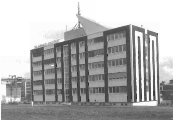
Figure 25 Installation of CdTe modules from First Solar LLC on an office building.
