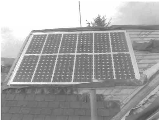
Figure 6 Flashing detail.
