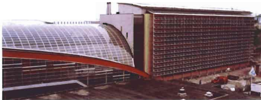
Figure 20 ECN, Buildings 31 and 42. © BEAR Architecten.
