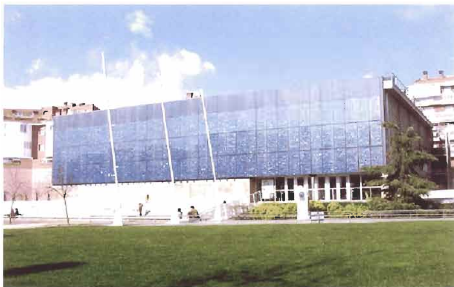
Figure 21 Pompeu Fabra Public Library. © Teulades i Façanes Multifuncionals.
