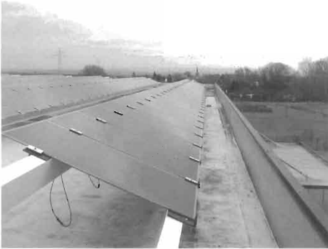
Figure 28 Close-up of mounting system on metal rafters for roof installation.
