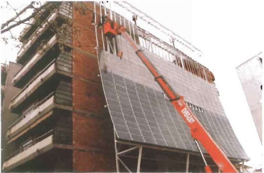
Figure 12 Installing an independent PV structure. © Teulades i Façanes Multifuncionals. Reprinted with permission.
