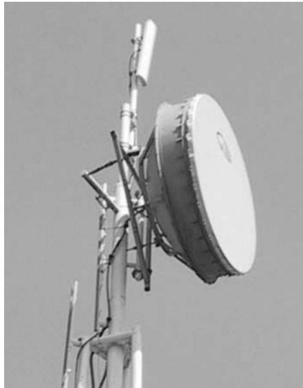
**Figure 6.23** Photo of a parabolic reflector ‘dish’ antenna with shroud and radome.
