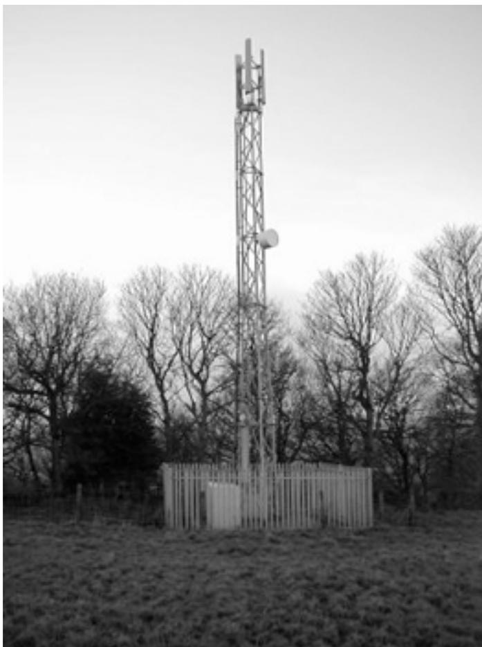
**Figure 6.12** *Tower-mounted sectored antennas (Courtesy of BT)*
