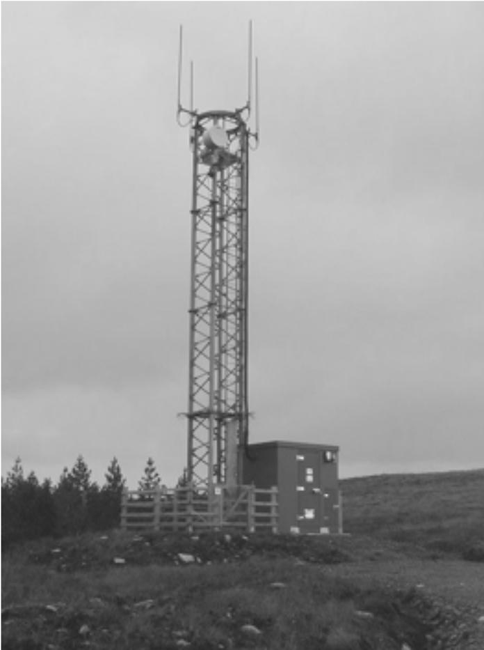
**Figure 6.13** *Tower mounted colinear antennas (Courtesy of BT)*
