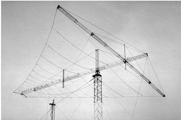
**Figure 2.6** *Horizontal log aperiodic (Courtesy Jaybeam Ltd)*
