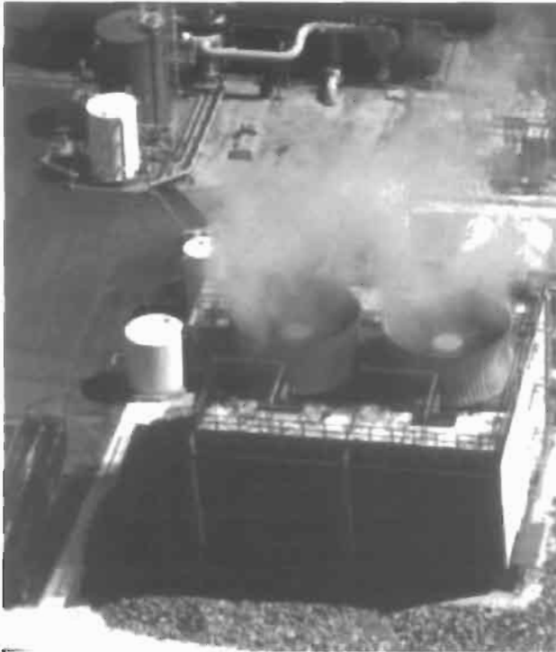
Figure 3.2 Vapour plume from cooling system at McKay Bay waste-to-energy facility, Tampa, Florida
