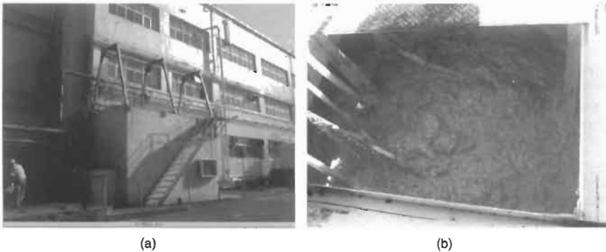
Figure 5.18 (a) Outside view of water tank and (b) MBR at N-food treatment plant
