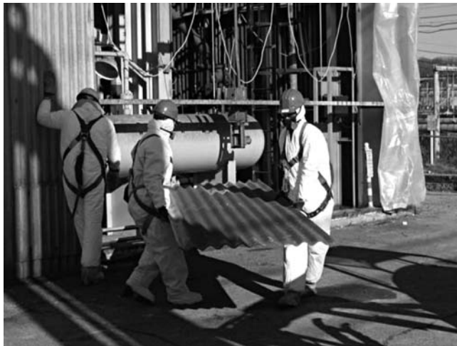
FIGURE 14.16 Decontamination workers fully dressed removing asbestos materials.
