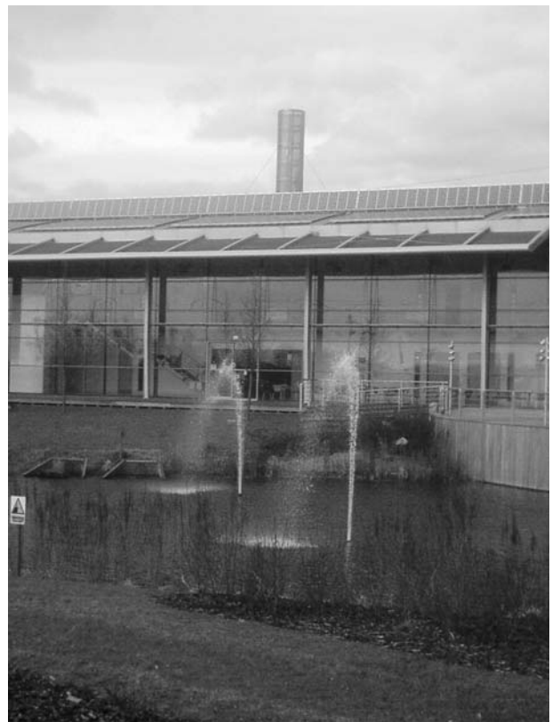
Figure 9-1 Photovoltaic-powered fountains enhance the CEME, U.K.
