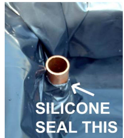
Close up of the Steam In pipe, use silicone caulk to seal this to the plastic.
