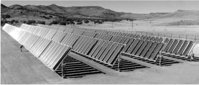
Figure 11.12 Entech 100-kW line-focus concentrator system in Fort Davis, Texas. Reproduced with permission by Entech, Inc.
