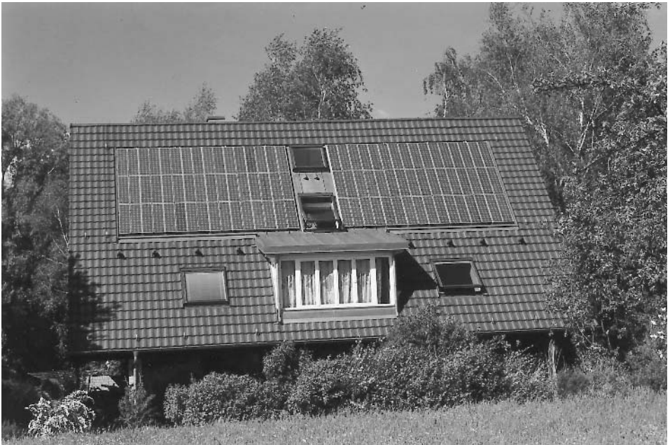
Figure 17.22 Grid-connected photovoltaic roof on a private house in Germany (Source: Fraunhofer ISE)
