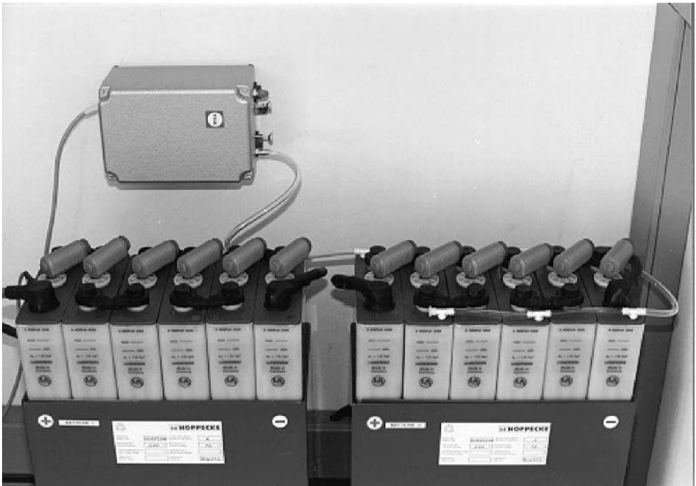
Figure 18.22 Flooded, tubular-plate battery ( 2 \times 240 Ah in parallel connection, 12 V) with gas recombinators for reduction of water loss through gassing and an electrolyte-stirring system to avoid acid stratification (only connected to the right hand unit), the membrane air pump is mounted on the wall, operation of the pump: twice a day for 15 min, (Picture courtesy Fraunhofer ISE)
