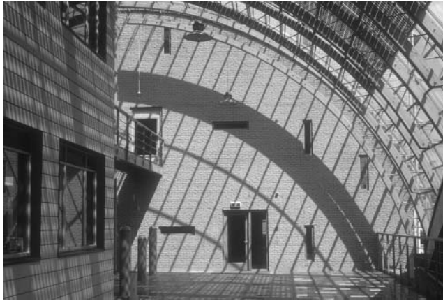
Figure 22.5 Interior view of the conservatory with integrated 43 kWp transparent BP solar modules in ECN Building 42 in Petten (NL). Reproduced with permission by BEAR Architecten T. Reijenga
