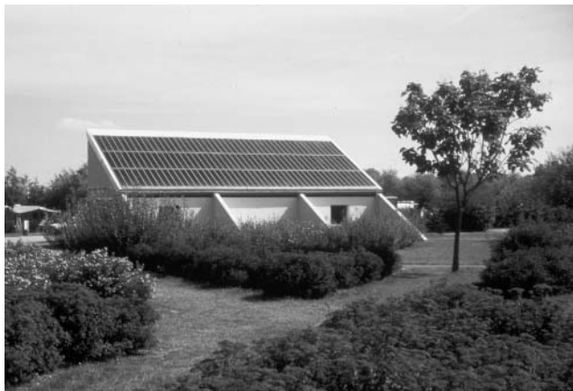
Figure 22.13 A naturally integrated PV system that is clearly part of the building. This system is located in Poitiers (FR). Reproduced with permission by ECN J. Beurskens
