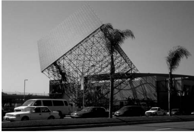
Figure 22.16 The cube at the Discovery Science Center in Santa Ana, Los Angeles, CA (USA). The 20 kWp PV system fits the gridula of this huge structure and there is harmony between the PV modules and the structure behind. Some 494 Thin-film Millienna photovoltaic modules from BP Solar were used on the solar cube. Reproduced from Eiffert P, Kiss G, Building-Integrated Photovoltaic Designs for Commercial and Institutional Structures – A Sourcebook for Architects , 48, 49, NREL, Golden, CO (2000) with permission by BEAR Architecten T. Reijenga [29]
