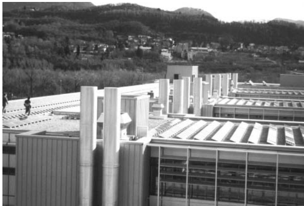
Figure 22.17 The 180 kWp Sofrel flat-roof system on the UBS Bank near Lugano (CH) matches the context of the roof, which fits between different installations, high-tech chimneys and the tight rhythm of the flat-roof PV system on the roof. Here the BIPV is mainly aesthetically and not physically integrated. Reproduced from Maycock P et al. , Building with Photovoltaics , 78–81, Ten Hagen & Stam, Den Haag (1995) with permission by UBS Switzerland [10]
