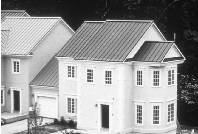
Figure 22.20 Houses at the National Research Home Park in Bowie, MA (USA) in historic style. The roofs are Unisolar standing-seam roofs with thin film (amorphous silicon). Reproduced with permission by NREL USA
