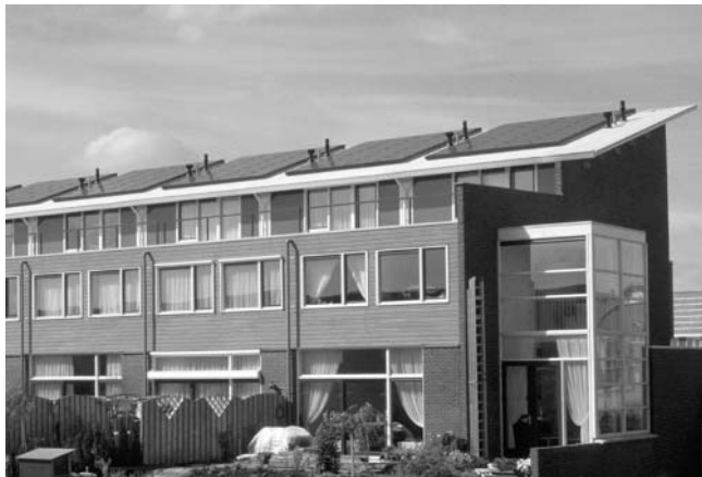
Figure 22.22 These houses in Amersfoort Nieuwland (NL) have a roof with a white foil on top. The architect chose a color contrasting with the color of the modules to show that the PV system is an addition to his design. Reproduced with permission by REMU J. van IJken
