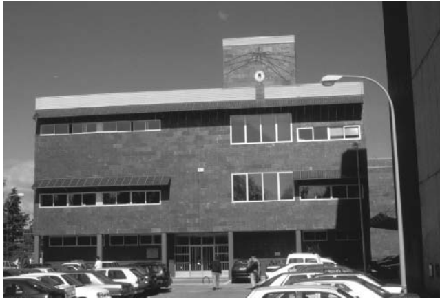
Figure 22.21 The IES building in Madrid (E) has a 6.6 kWp PV system that was added shortly after the building was finished. The modules are mounted on the façade above the windows and keep out the sun. Reproduced with permission by BEAR Architecten T. Reijenga
