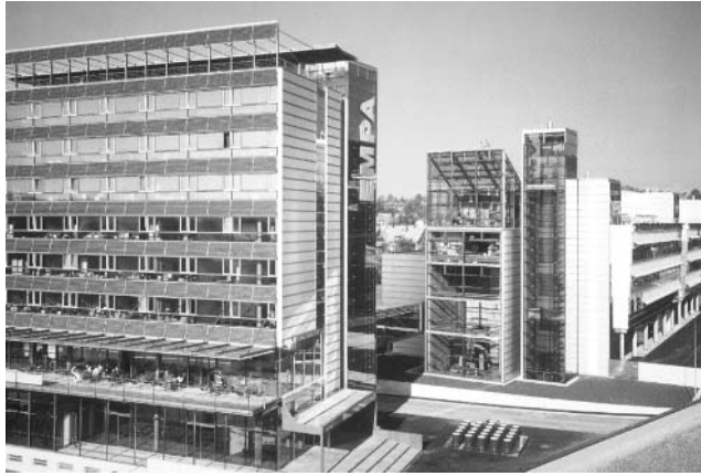
Figure 22.23 The architect integrated the (in total 49 kWp) PV modules into the facades above the windows and produced a combination with the roller blinds. The EMPA office building is located in Sankt Gallen (CH). Reproduced with permission by Electrowatt Eng. Services
