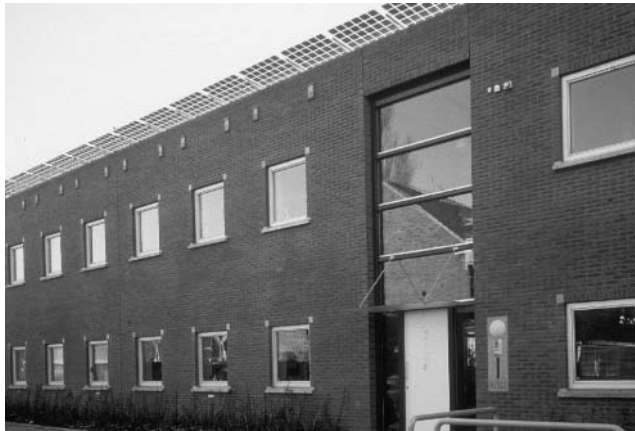
Figure 22.24 In this office building in Gouda (NL), the 6.2 kWp PV system is mounted on top of the façade as a canopy that protects the wall. The architect’s intention was to show the PV system to his clients when they visit the office. Reproduced with permission by BEAR Architecten T. Reijenga
