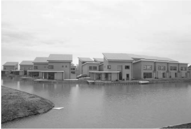
Figure 22.25 The dwellings at the 5 MW project in the HAL district of Langedijk (NL) have a large PV roof without any perforations. This strengthens the architectural expression of the roof design. Each roof includes a 5.1 kWp BP Solarex PV system. Reproduced with permission by BEAR Architecten M. van Kerckhoven
